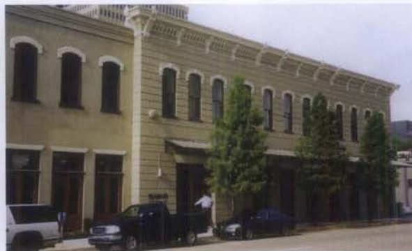
Figure 28. A small addition (left) was constructed when this 1880s train station was converted for office use. The paired doors with transoms and arched windows on the compatible addition reflect, but do not replicate, the historic building (right).
