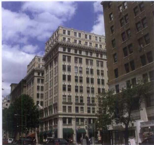
Figure 19. The upper two floors of this early-20th century office building were part of the original design, but were not built. During rehabilitation, the two stories were finally constructed. This treatment does not meet the Standards because the addition has given the building an appearance it never had historically.
