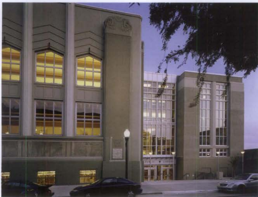
Figure 1. The addition to the right with its connecting hyphen is compatible with the Collegiate Gothic-style library. The addition is set back from the front of the library and uses the same materials and a simplified design that references, but does not copy, the historic building. Photo: David Wakely Photography.
