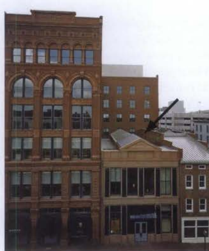
Figure 21. Both wings of this historic L-shaped building (top), which fronts on two city streets, adjoined vacant lots. A two-story addition was constructed on one lot (above, left) and a six-story addition was built on the other (above, right). Like the historic building, which has two different facades, the compatible new additions are also different and appear to be separate structures rather than part of the historic building.
