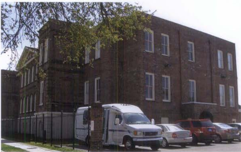
Figure 9. A simple, brick stair tower replaced two non-historic additions at the rear of this 1879 school building when it was rehabilitated as a women's and children's shelter. The addition is set back and it is not visible from the front of the school.
