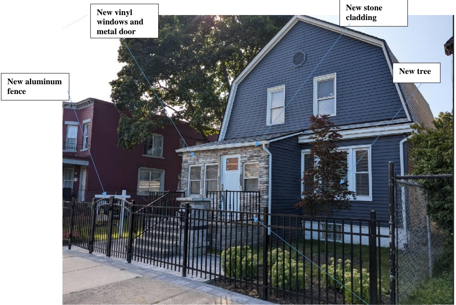
4081 Porter. Photo by staff taken in August 2024 after unapproved work.
