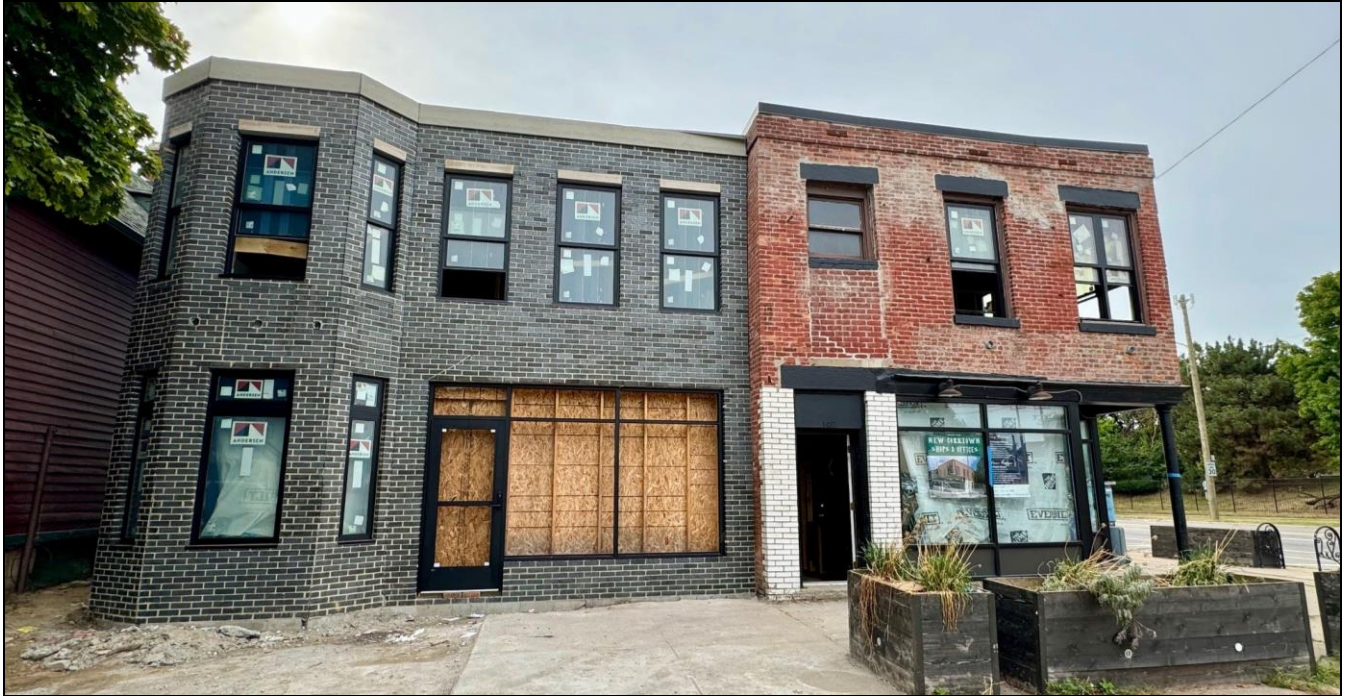
1451 Bagley façade. Staff photo, September 2024.
