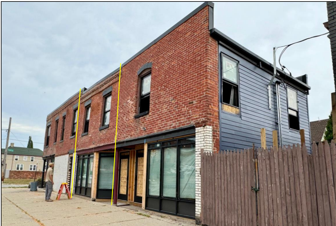
Trumbull elevation looking northeast. Staff photo, September 2024. The building has a registered address of 1451 Bagley, but the section/storefront subject to this application is identified with the address of 1550 Trumbull. (area between the yellow lines).
