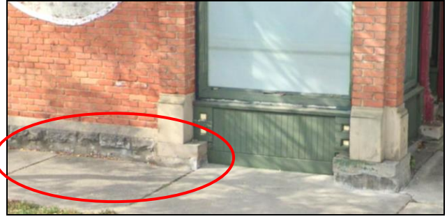
Consistent stone base at 1401 Bagley.
