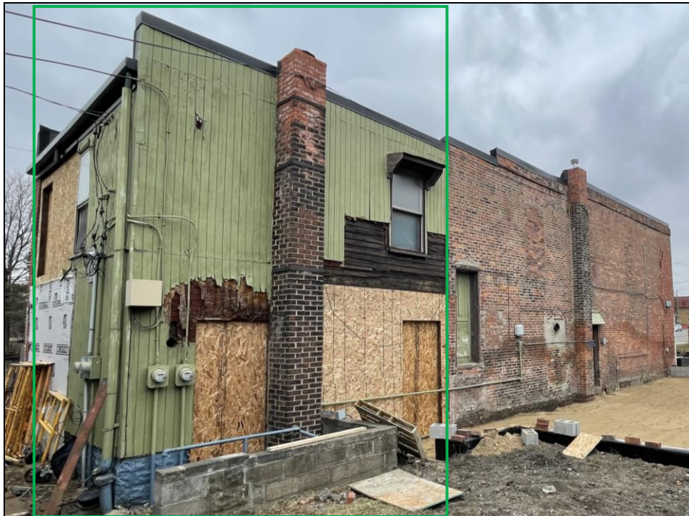
View of east wall in early 2024. Photo provided by building owner.
