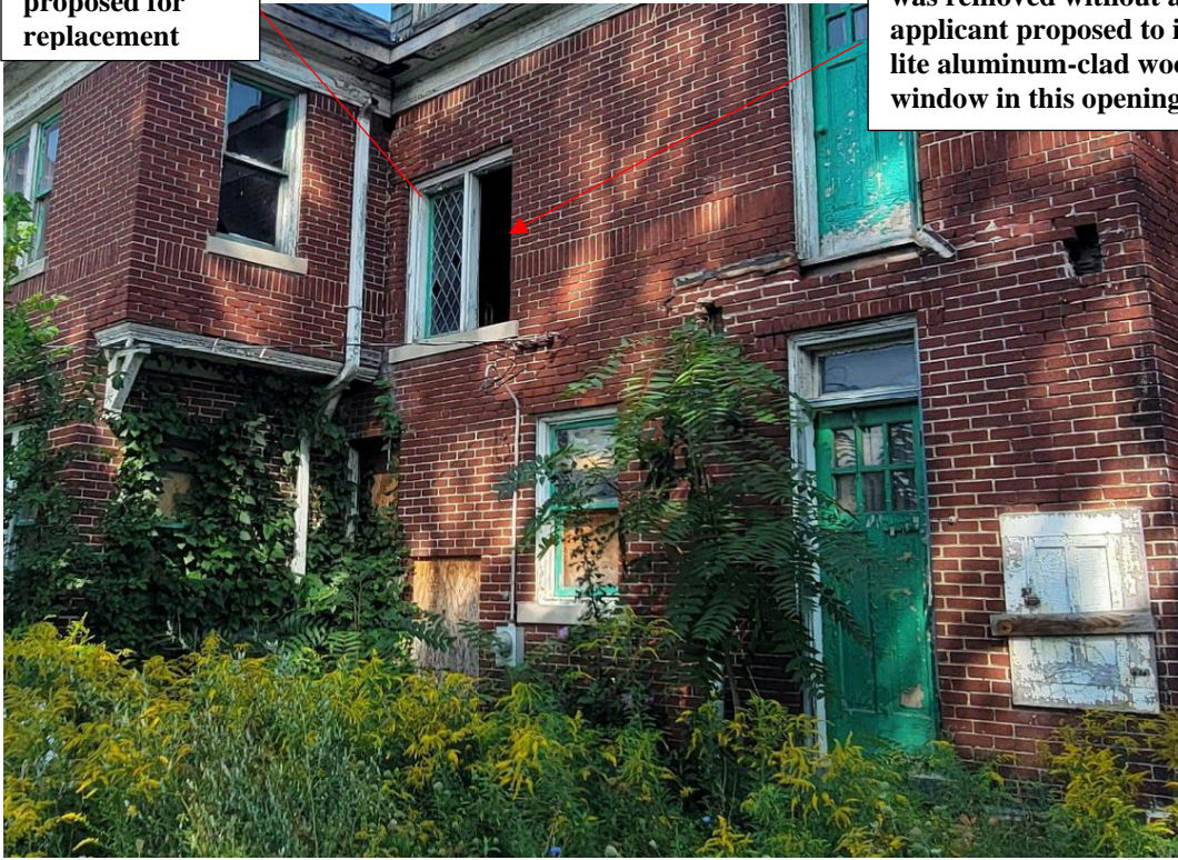
Rear wall, current appearance. Photo by applicant
