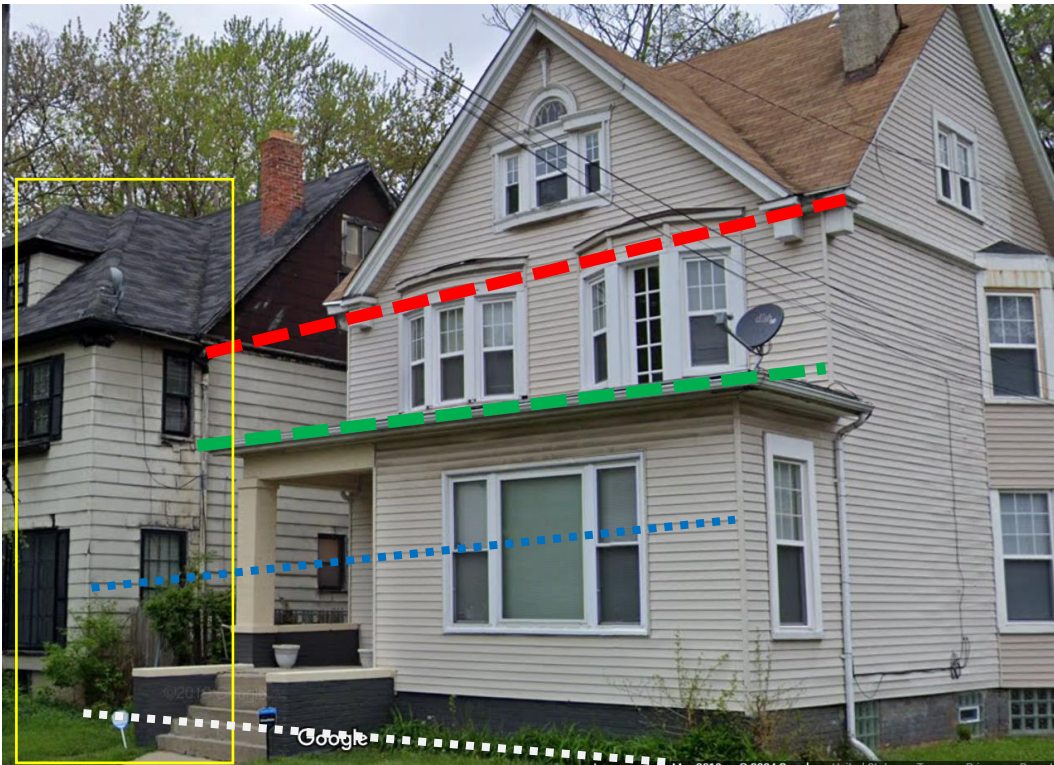
7873 Van Dyke Place (left) and 7881 Van Dyke Place (right). Per the above Sanborn Map from 1915, both houses were similar in plan, form, and setback. By 1951 the porch at 7874 Van Dyke Place had been infilled and second story added (see area outlined in yellow). The red dashed line indicates matching gable end/peaks, the green dashed line indicates matching south gable edges, the dashed blue line indicates matching front/south wall face, and the white dashed line indicates matching south foundation wall. Face/setback, Source, 2022 Google Streetview
