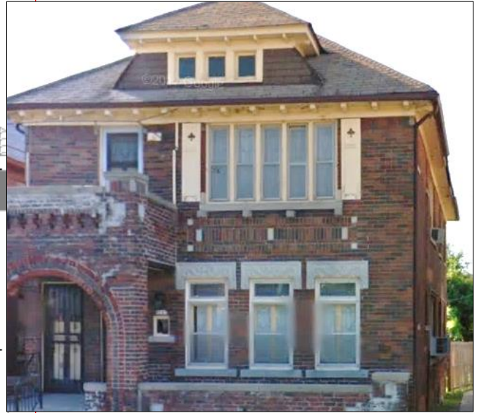
August 2011 Google street view photo. The leaded glass casement windows at the first and second floor are disguised due to the installation of double-hung storm windows.
