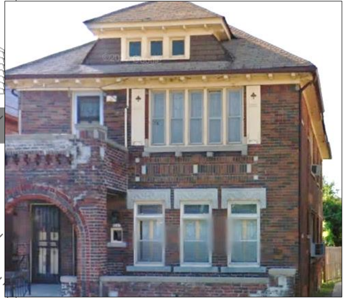
August 2011 Google street view photo. The leaded glass casement windows at the first and second floor are disguised due to the installation of double-hung storm windows.
