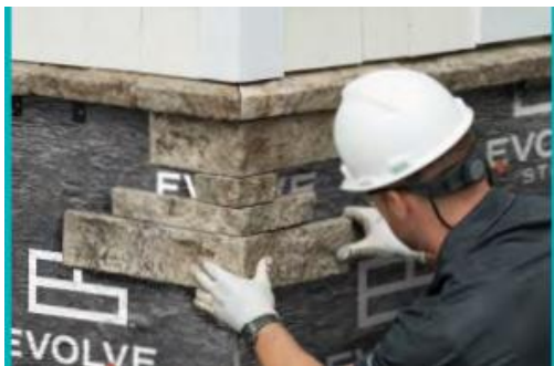
Evolve Stone veneer image (from product brochure) showing depth of material and thickness of joints.
