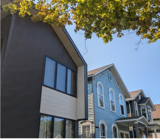
Three Corktown buildings on Wabash that demonstrate how projecting eaves (typical of the district) create a sense of depth. On the twenty-first-century building (left), a sense of verticality is enhanced by corrugated siding and a continuation of the eave down the side of the façade. On the historic buildings (center and right), verticality, depth, and texture, are created by window hoods, projecting gables, and a bay window. September 2024 photo by staff.
