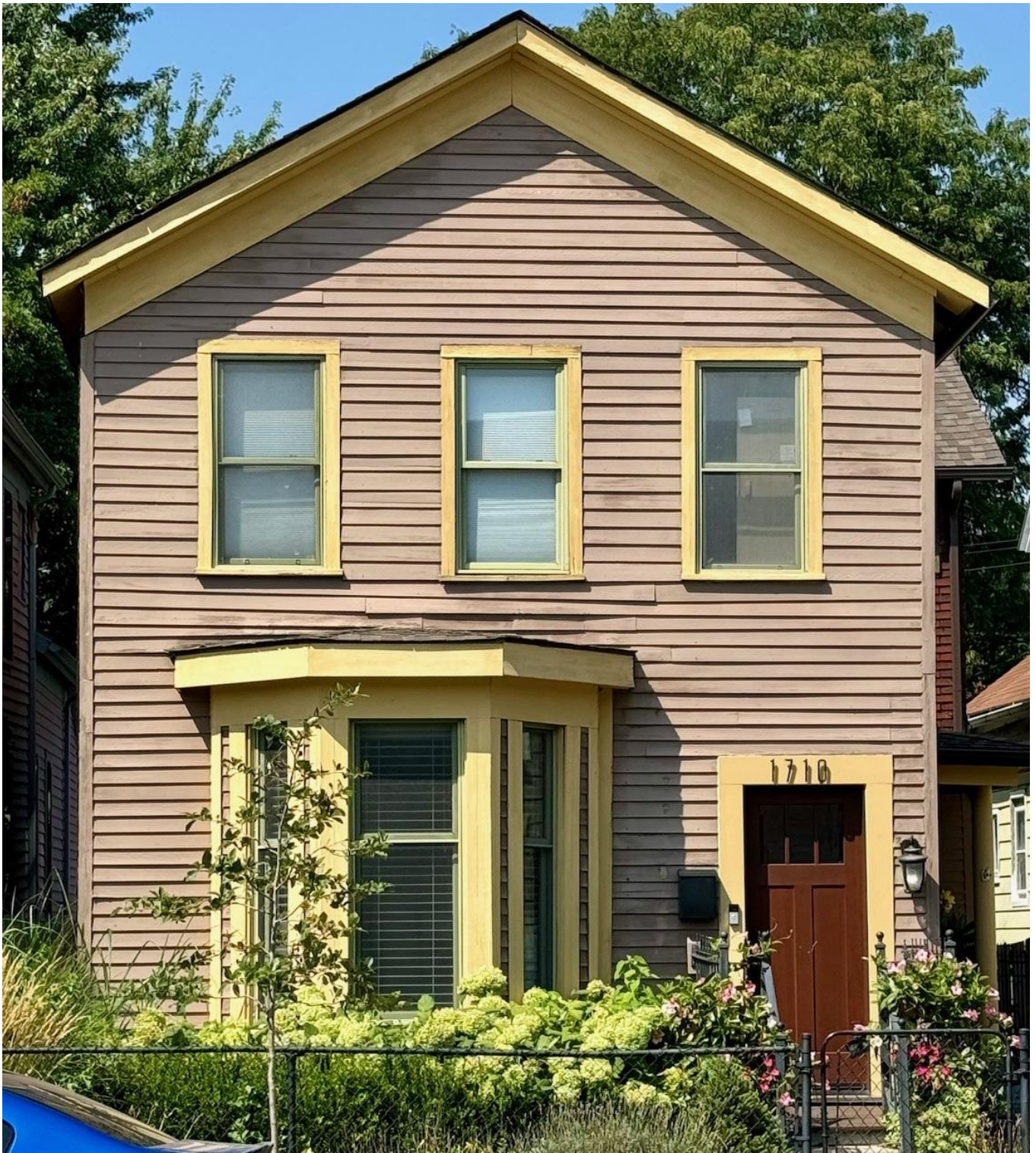
Existing conditions on facade of house, August 2024. Staff photo.
