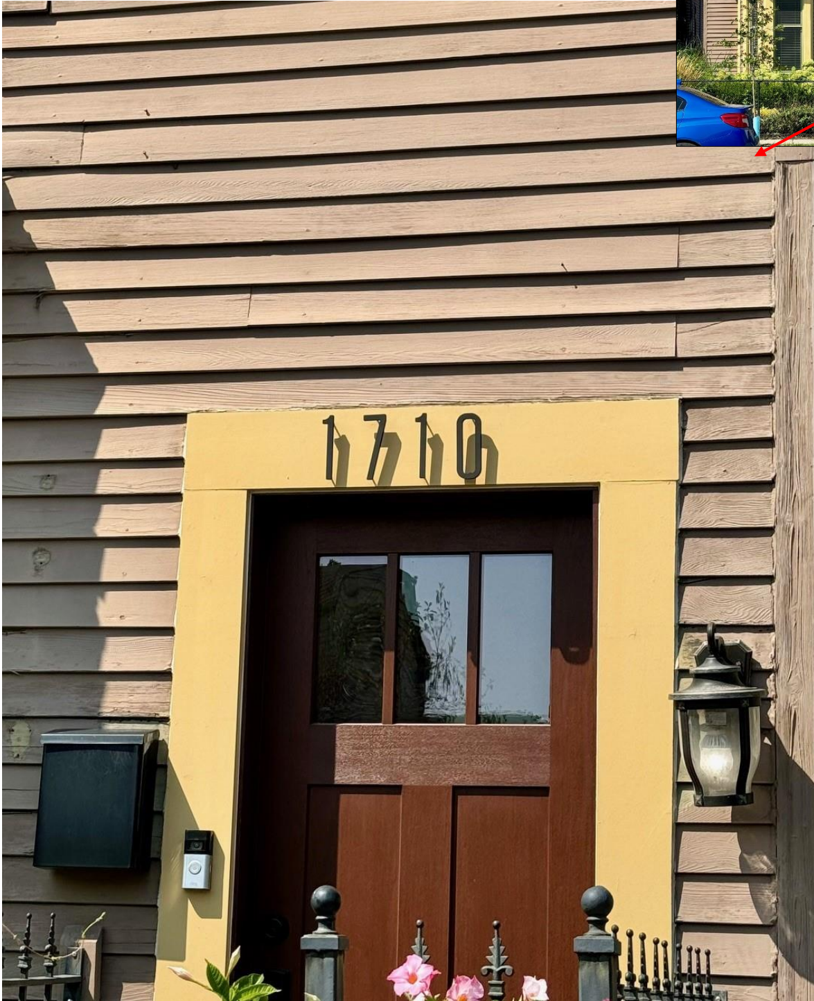
Existing conditions of siding at front entrance, August 2024. Staff photo. The lap siding was installed with different length pieces, creating visible seams.
