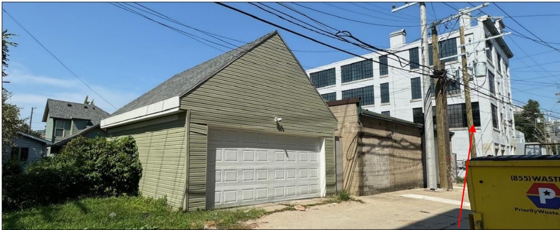
This photo, looking northeast from the alley, shows the close proximity of the Kaul Glove Company building. Erected in 1917 for the Robert Keller Ink Company, the HDC reviewed an application for the building's rehabilitation in 2021. It is now used as office space for multiple companies.
