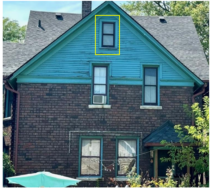
Rear – east wall
