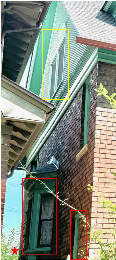
Side – North wall
