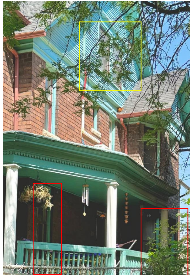
Side – South wall
