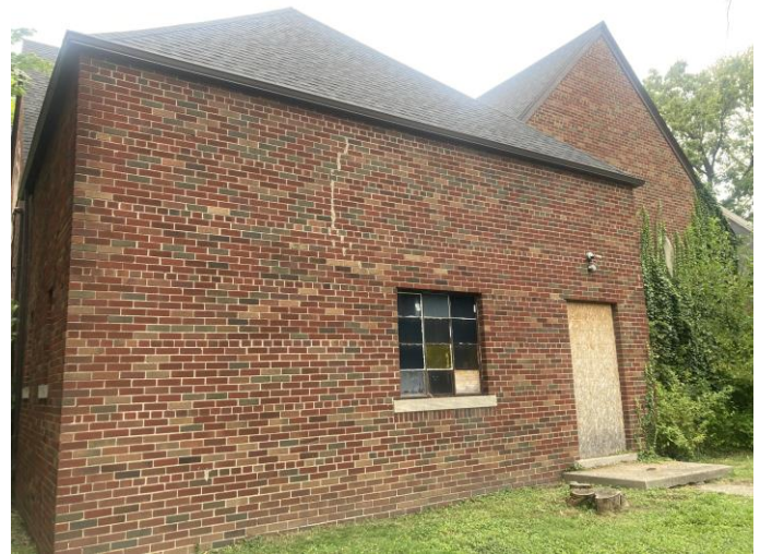
This window at the rear of the sanctuary’s south wall is proposed to be replaced with a fixed aluminum clad unit.
