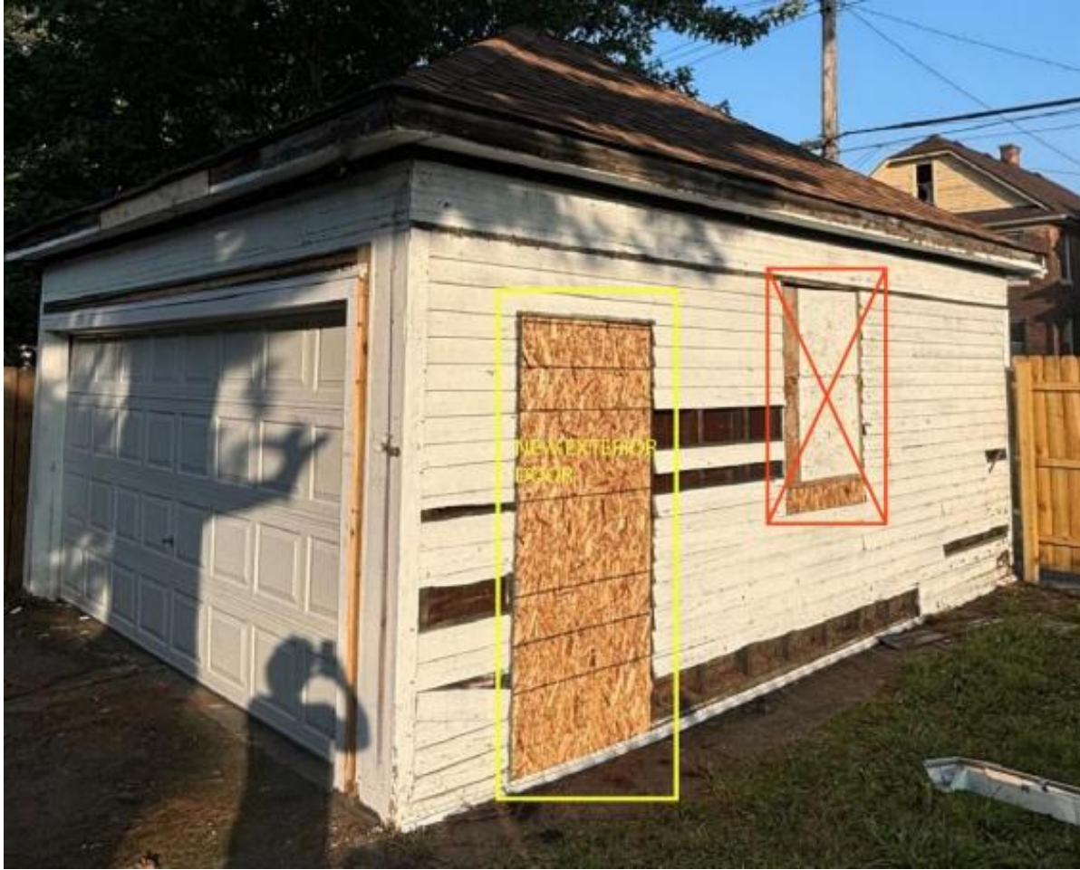
1667 Edison, garage, current appearance. Photo provided by applicant
