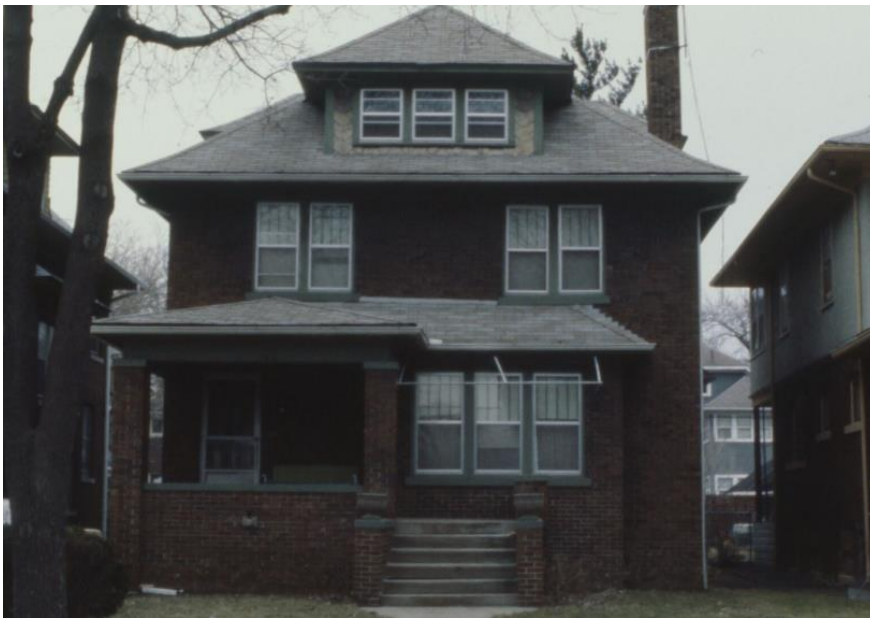
1667 Edison, designation slide taken by the HDAB in 1980. Note that the property has aluminum storm windows. However, all of the original/historic wood windows remained intact behind the storms
