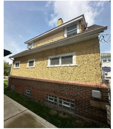
Site Photo 4, by Applicant, 2024: (West) side elevation showing vinyl and glass block windows. (Image is slightly skewed by applicant to fit this tight location in one photo.)
