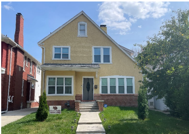
Site Photo 1, by Staff Aug. 22, 2024: (North) front showing replaced vinyl windows, altered porch and landscape.
