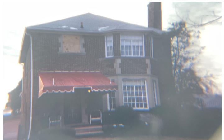
Site Photo 2, designation slide 1999: (North) front showing original steel sash casements with true divided light.
