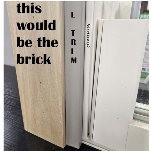
Figure 9, by Applicant: This is a mock-up to illustrate the use of the "L-Trim" aluminum coil stock that would be set between the window and brick opening.
