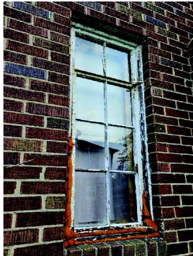
Figures 4&5, by applicant 2024: Window #104, west side, showing casement window condition with foam applied to exterior.
