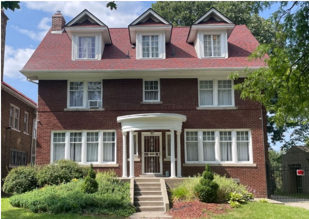
Site Photo 1, by Staff Aug. 22, 2024: (South) front side showing original wood windows still in place.
