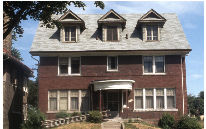
Site Photo 2, designation photo 1974: (South) front side showing original wood, double-hung windows with true divided light.
