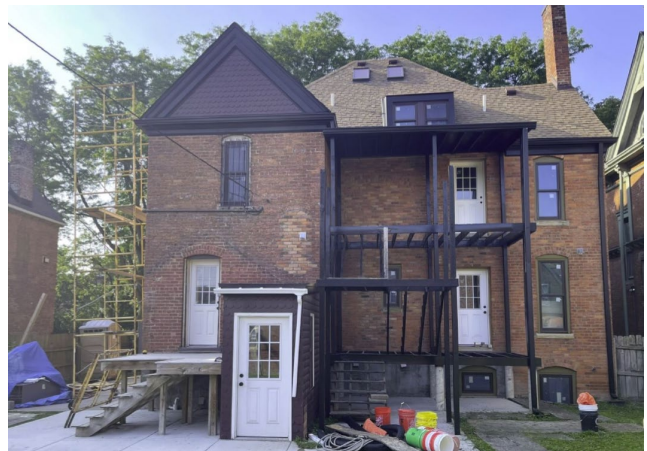
Site Photo 2, by Applicant July 2024: (South) rear elevation showing current conditions.
