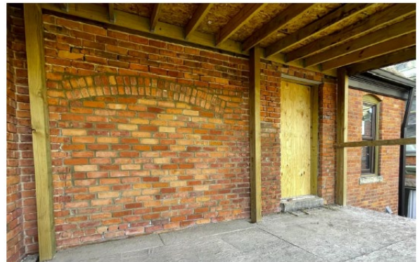
Site Photo 3, by Applicant, date unknown: (South) rear elevation, showing original arched brick detailing over door and window openings.
