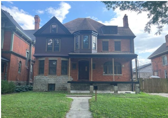
Site Photo 1, by Staff July 25, 2024: (North) front elevation showing current conditions.
