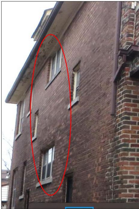
3747 Tyler, 2018 east elevation. Triple, equally proportioned mulled window frames are visible.
