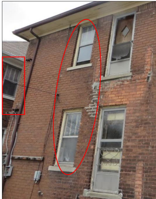
3747 Tyler, 2018 rear elevation. Vertical upper sash pattern is visible at both properties. (3755 Tyler partially shown.)
