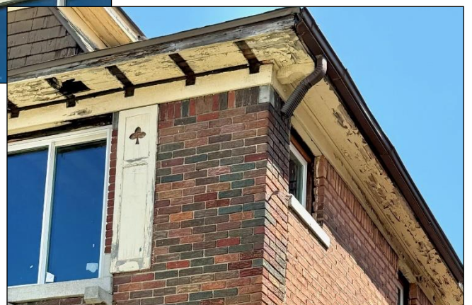
Left and below: 2024 staff photos showing existing conditions at the second floor eaves and the intact historic design at the dormer eaves.
