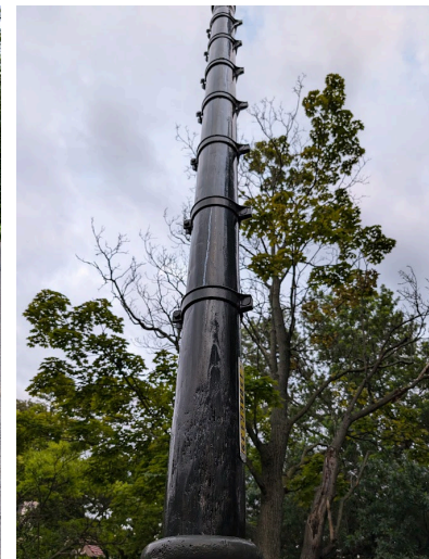
Original 110-year old PLC pole, restored and reinstalled in Indian Village HD. Note cast iron base, wood shaft, foot pegs.
