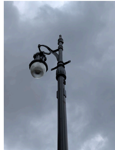
Here is an example of a reproduction steel PLC pole, one of many installed in recent years downtown. Note modern construction (two-halved base, steel pole with no footpegs) in comparison with the cast iron base and wood shaft on an original pole pictured below.
