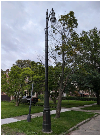
Original 110-year old PLC pole, restored and reinstalled in Indian Village HD. Note cast iron base, wood shaft, foot pegs.
