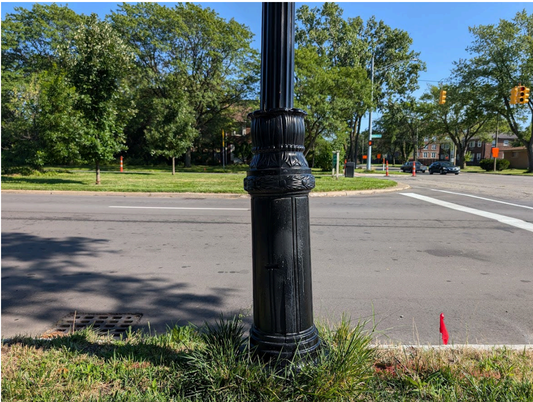
Detail view of a fiberglass pole along Oakman. Note dislocated base leaning to the left, as well as the machined “historic” details attempting to portray a traditional appearance with no historic connection to the Oakman Boulevard Historic District. The dominant expression of these poles are gaudy and cheap. Staff photo, August 7, 2024.
