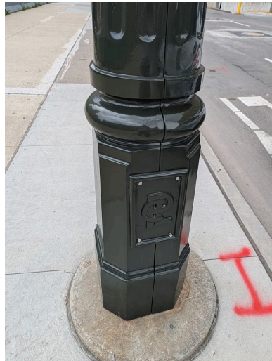
Here is an example of a reproduction steel PLC pole, one of many installed in recent years downtown. Note modern construction (two-halved base, steel pole with no footpegs) in comparison with the cast iron base and wood shaft on an original pole pictured below.
