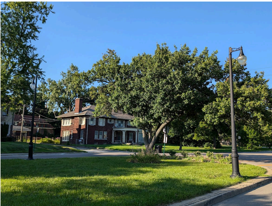
Existing fiberglass poles flanking Chicago Boulevard in Boston-Edison Historic District. Some of the plastic luminaires on these poles have been replaced with smaller globes, contributing to a chaotic appearance, Staff photo, April 7, 2024.
