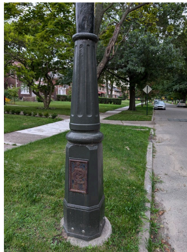
Original 110-year old PLC pole, restored and reinstalled in Indian Village HD. Note cast iron base, wood shaft, foot pegs.
