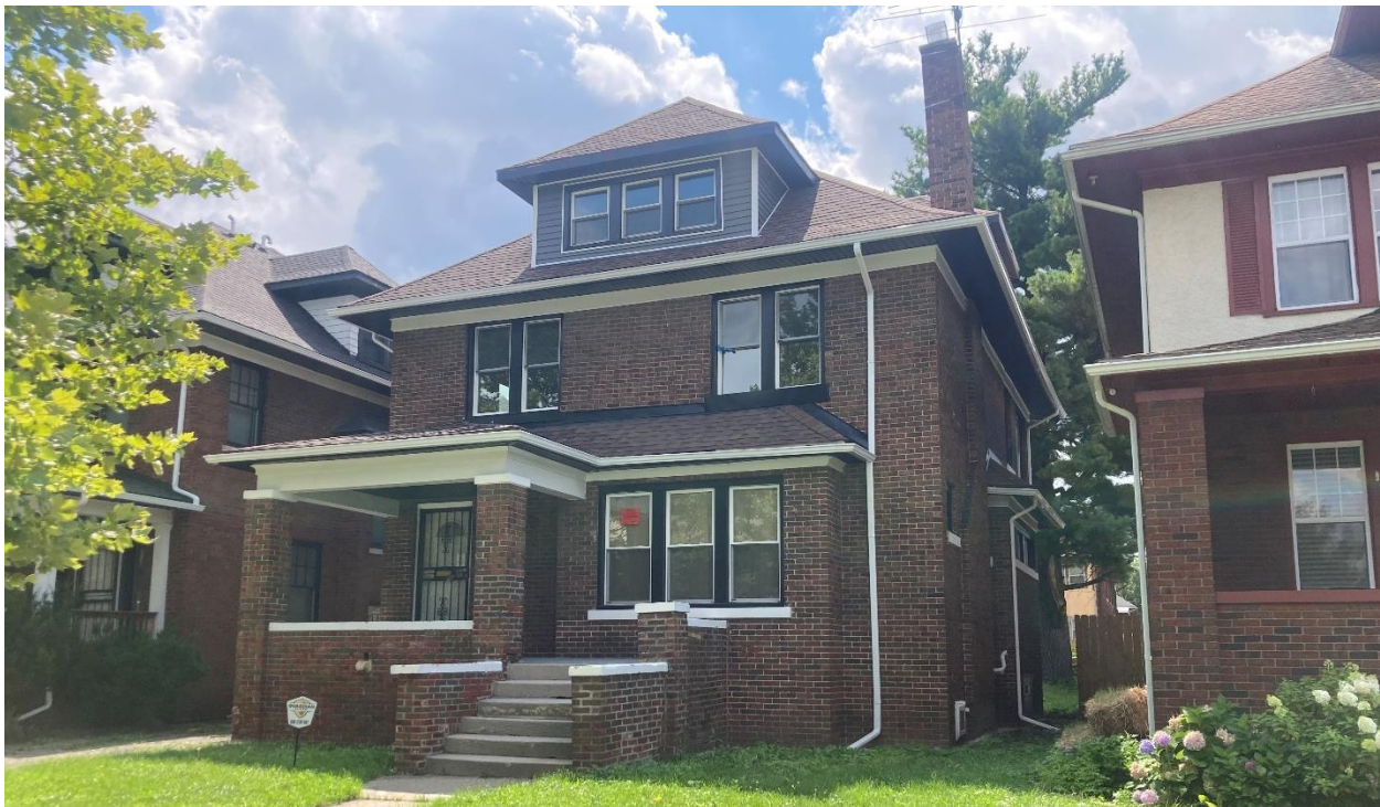
1667 Edison, current appearance. Photo taken by HDC staff on 7/25/2024
