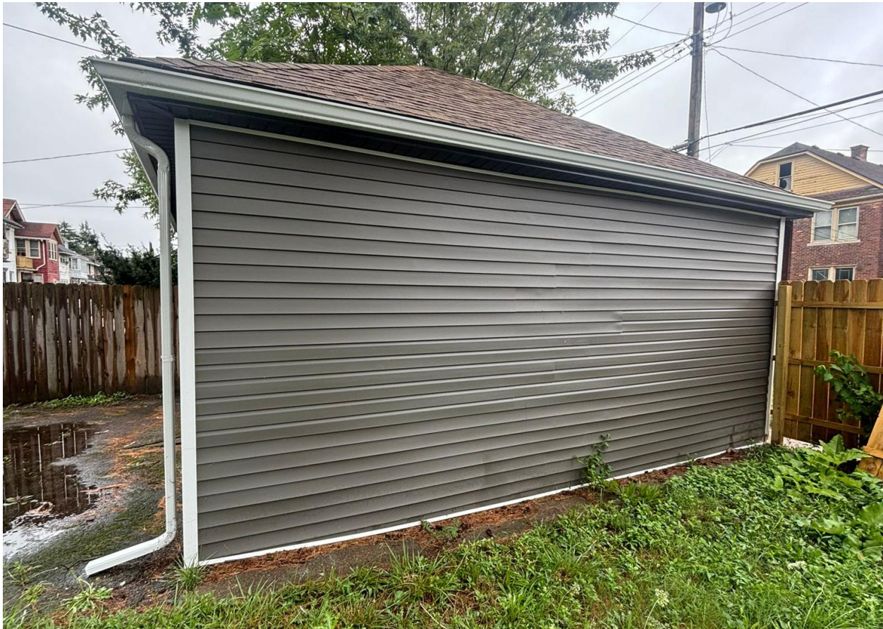
1667 Edison, garage. Photo provided by applicant
