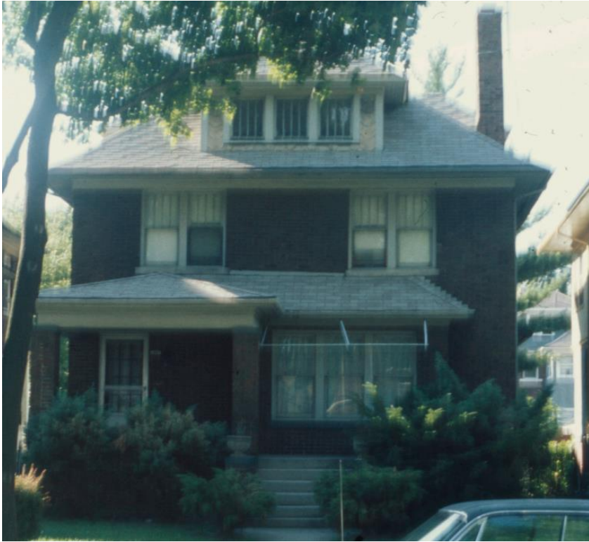
1667 Edison, designation slide, taken by the HDAB in 1974
