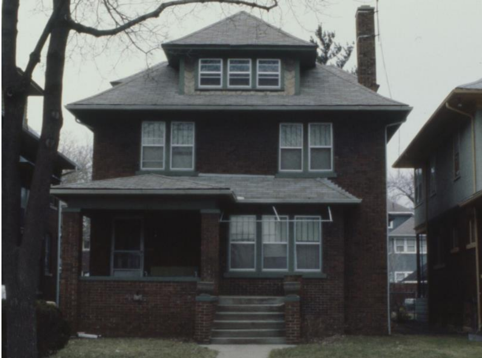
1667 Edison, designation slide taken by the HDAB in 1980. Note that the property has aluminum storm windows. However, all of the original/historic wood windows remained intact behind the storms
