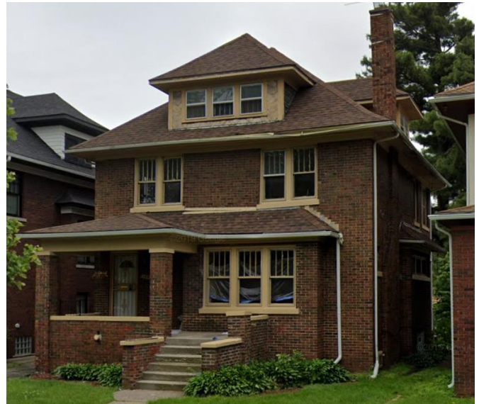
Google Streetview images, taken in 2016. Note that the attic/dormer 4-light wood windows are present but covered on the exterior by storm windows. Also, note that windows at the side elevation appear to be the same 4/1 type which were present at the front façade.
