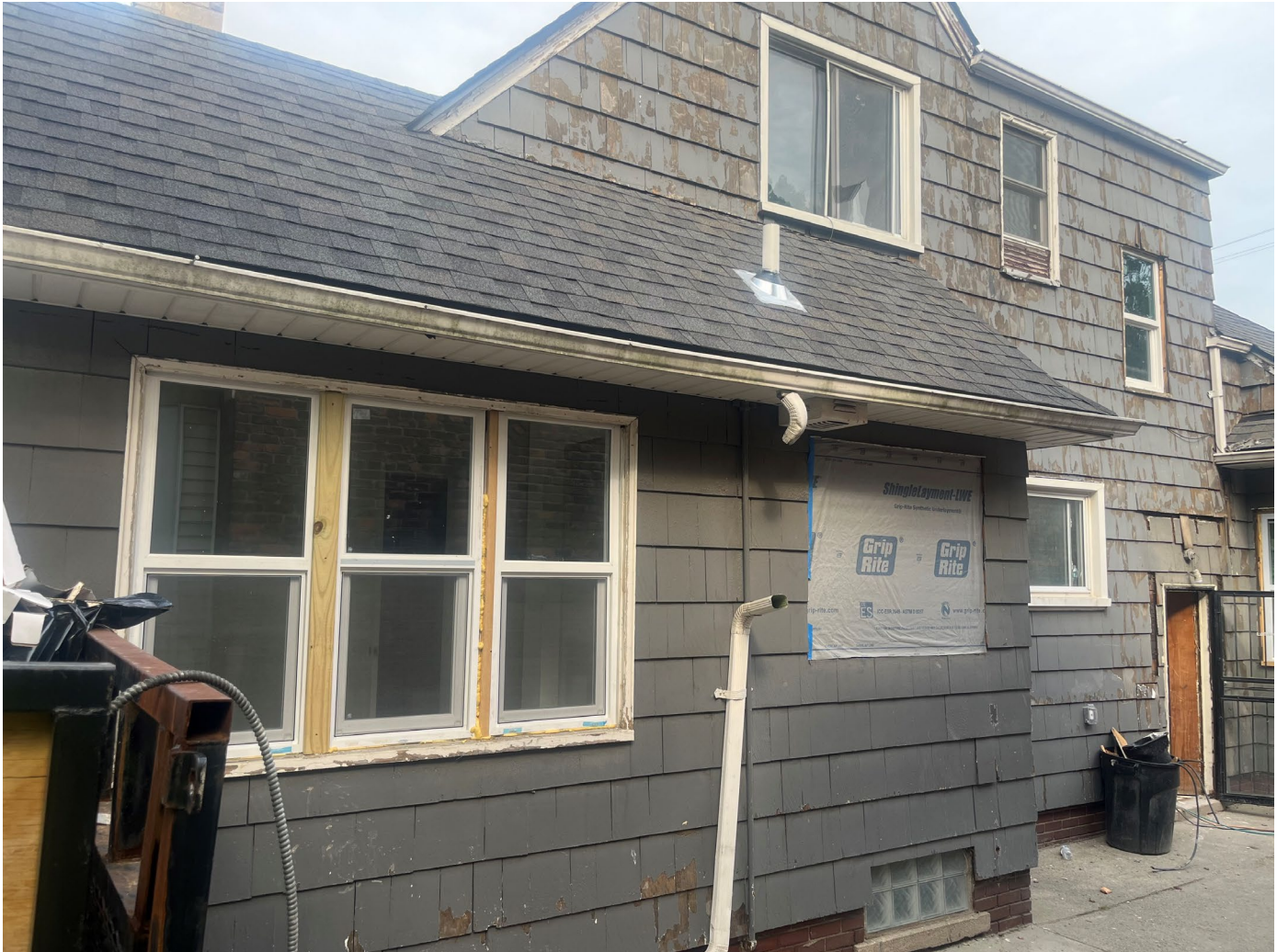
Figure 3: Image showing east side of dwelling with new windows and an infilled window opening.
