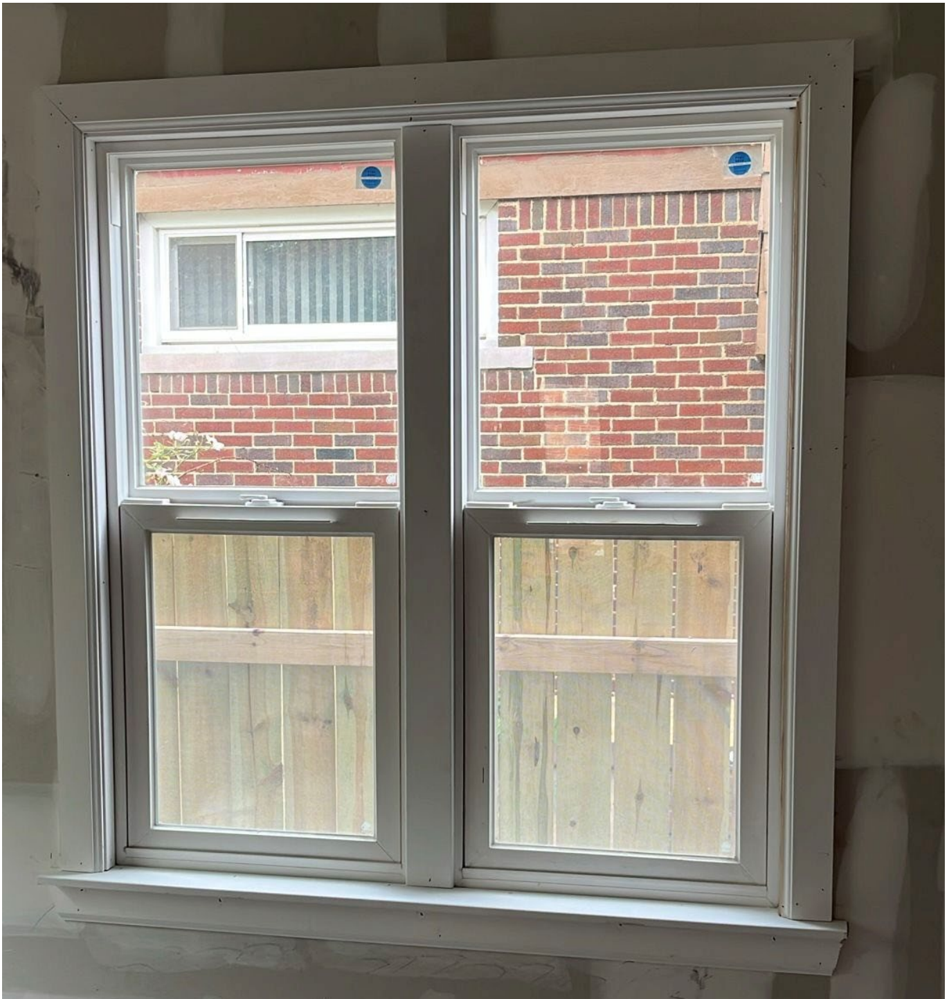
Figure 6: View of new windows from interior of the dwelling.
