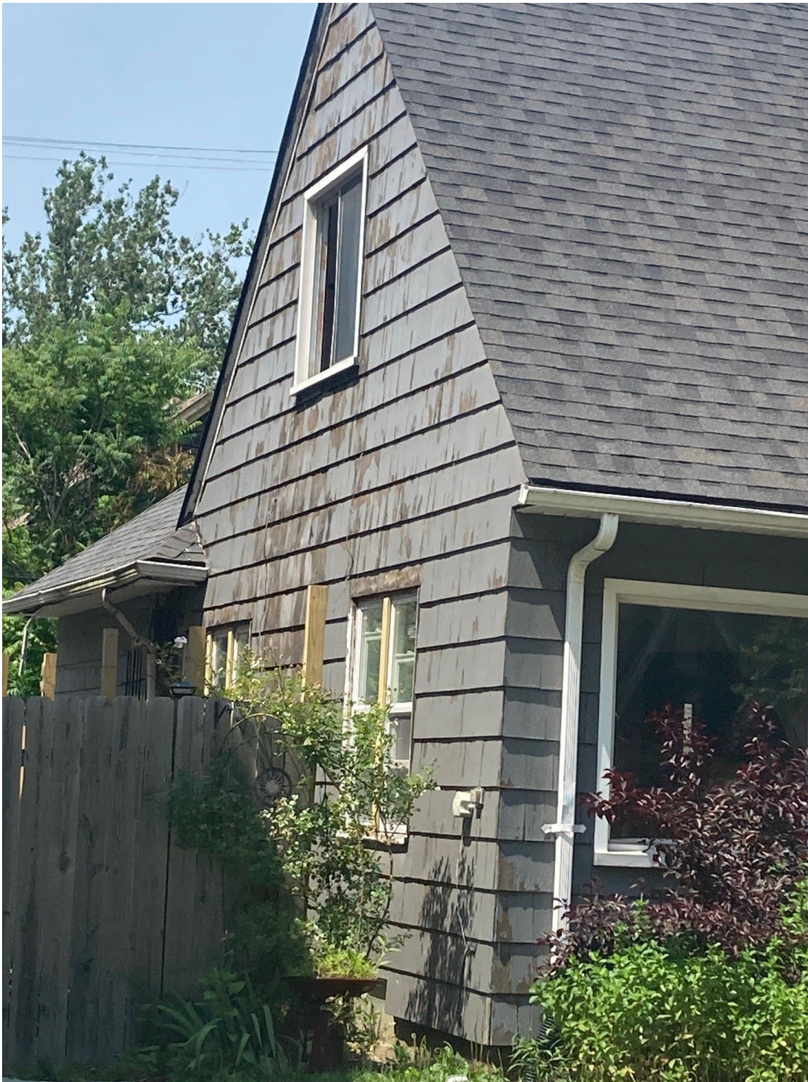
Figure 5: View of replacement windows on west side of property.
