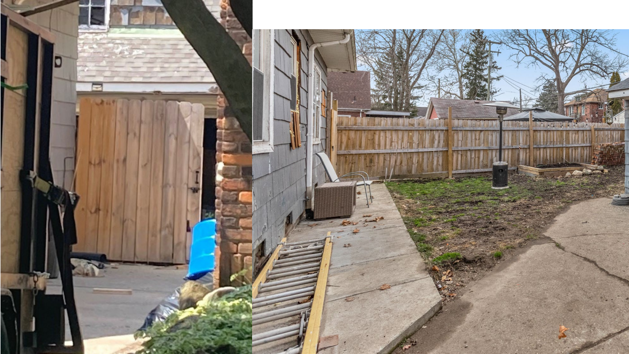
Figure 9: Images showing the fence and gates as installed.
