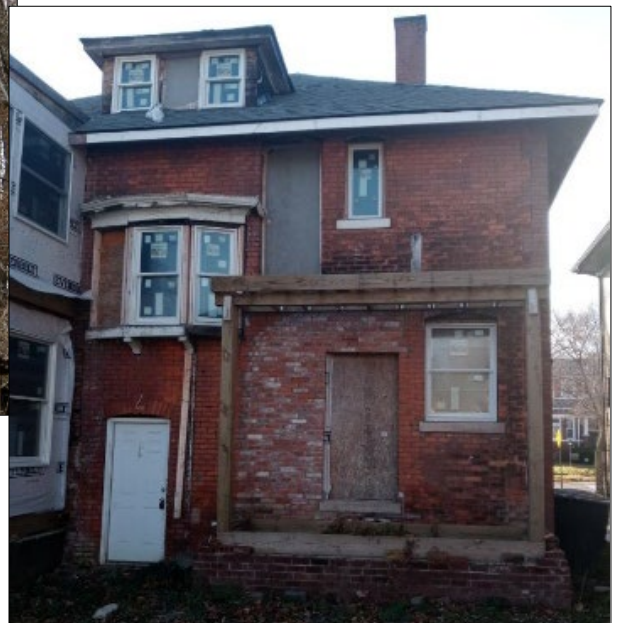
2020 photo provided with application for new gutters.
