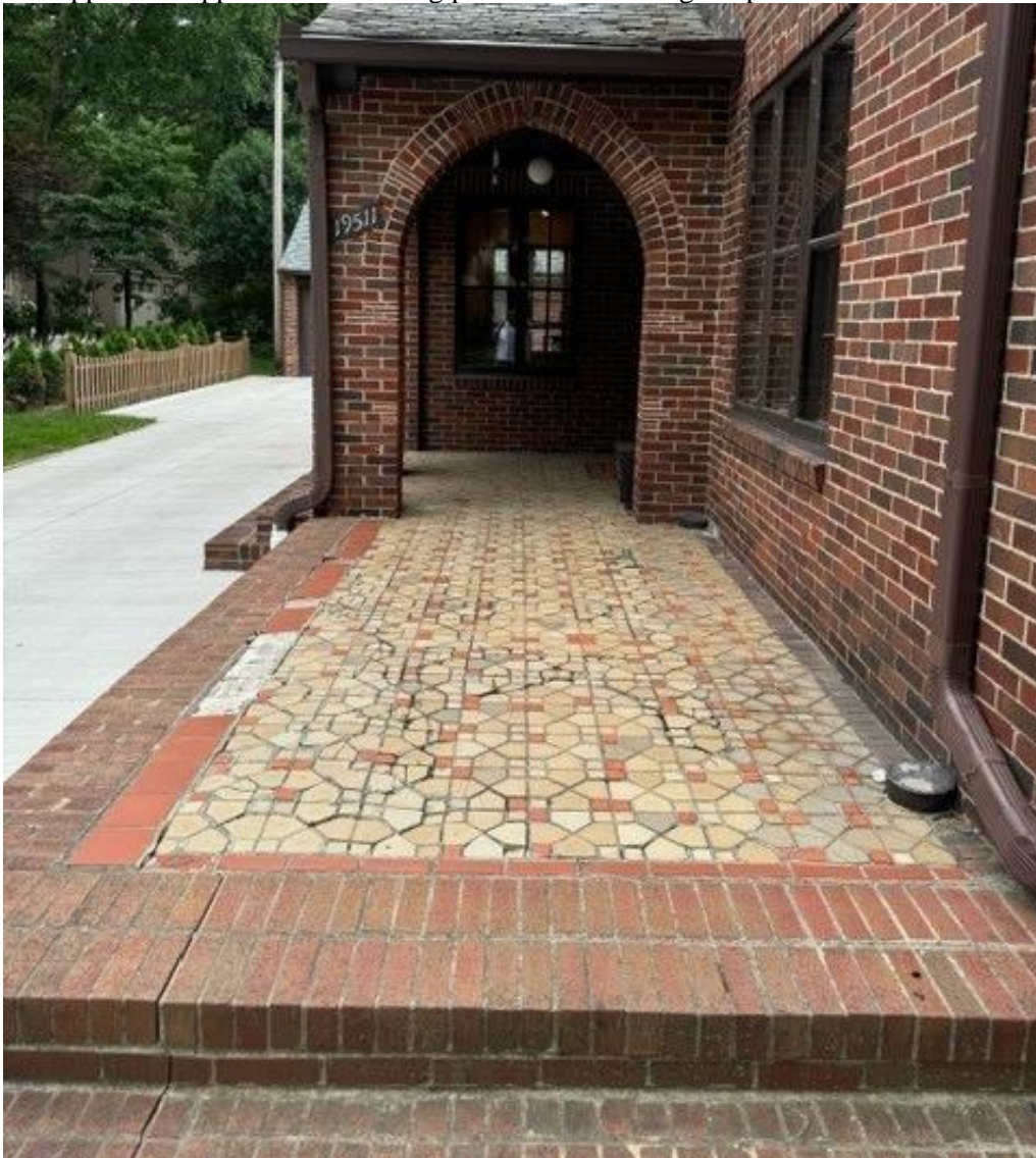
Applicant photo. View from steps at front walkway. Three different materials are used to edge the tile floor: square clay or quarry tiles at the west perimeter, narrow rectangular tiles at the northern perimeter, and a rowlock course of dark colored bricks at the western perimeter adjacent the house.
