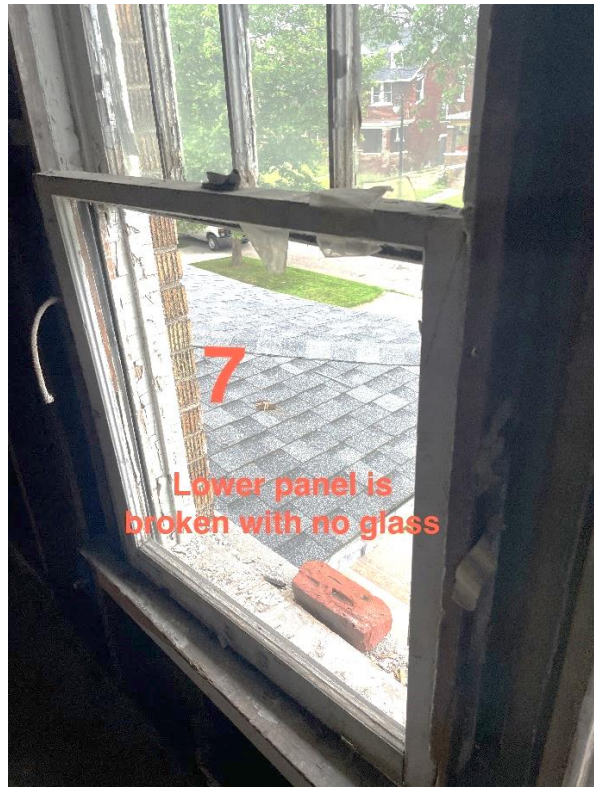
The glass in the bottom sash (6) may need to be replaced and new glass is needed for (7).
