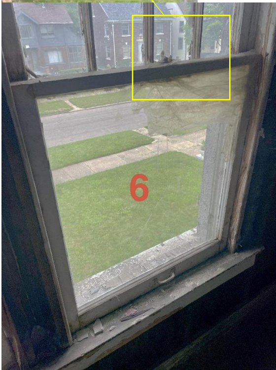
The glass in the bottom sash (6) may need to be replaced and new glass is needed for (7).
