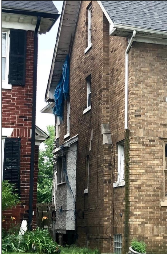
East-side wall. Staff photo, June 21, 2024.
