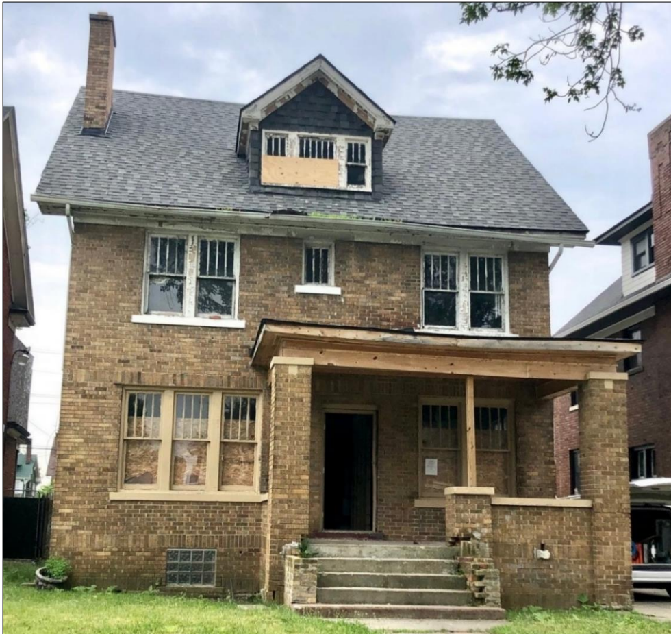
Façade, north-facing wall. Staff photo, June 21, 2024.
