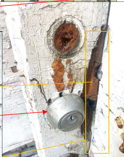
Left – red box identifies cracked frame. Above: orange box and arrows to adjacent photo show dimensional views of missing sections of door frame. Bottom left: additional section of missing door frame.
