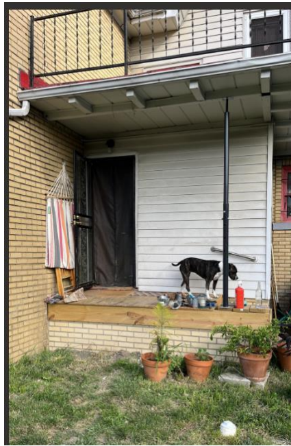
Rear porch. Condition prior to unapproved repair (left) and current condition showing new brick, wood decking, and temporary support (right). Photos provided by applicant
