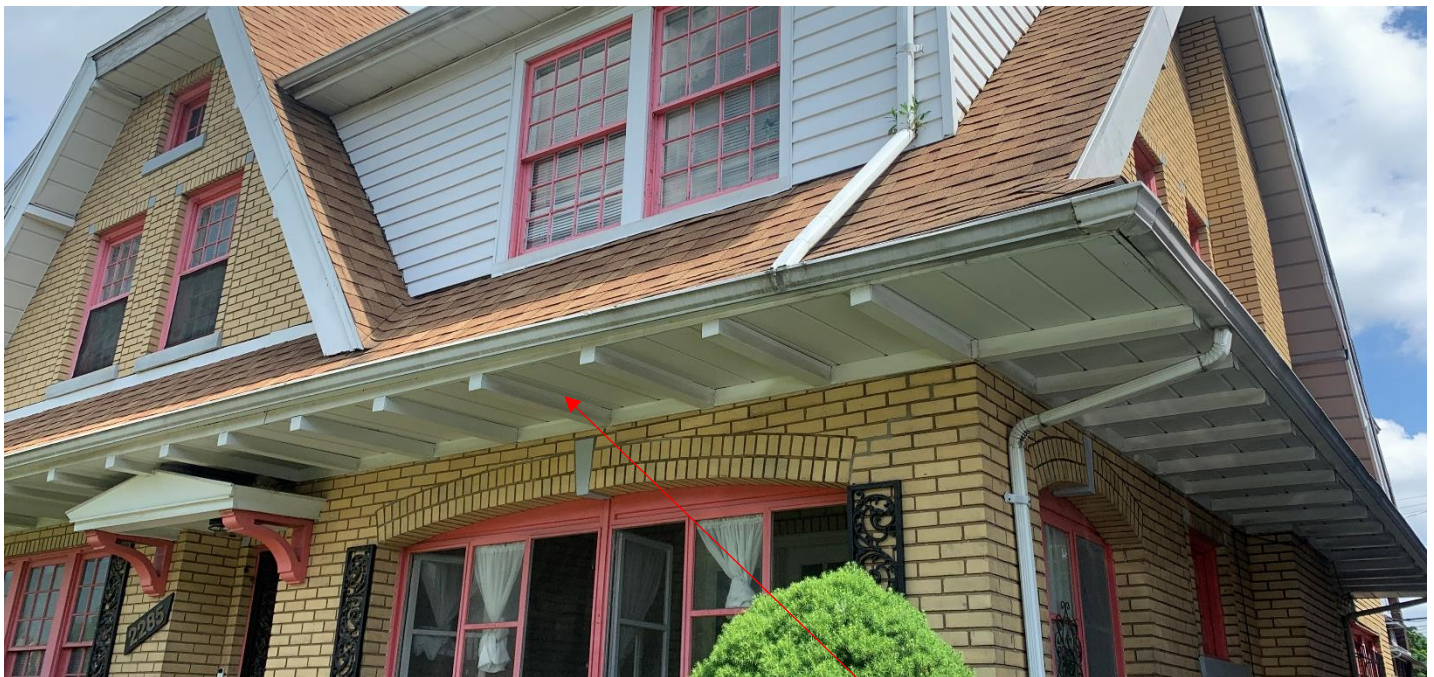
Photo by applicant. Showing brackets in the eaves, currently wrapped in aluminum
