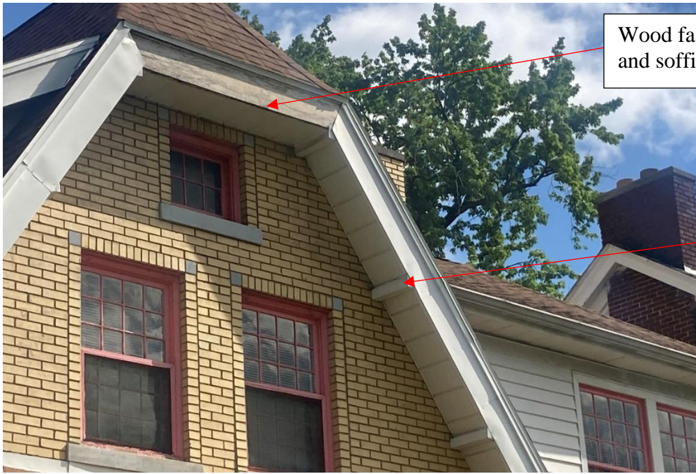
Staff photo, taken on 5/29/2024. Facing front elevation gable end. Note that an area of the original wood fascia is visible after a portion of the aluminum wrapping has fallen off. Also note brackets in the eaves, currently wrapped in aluminum.
