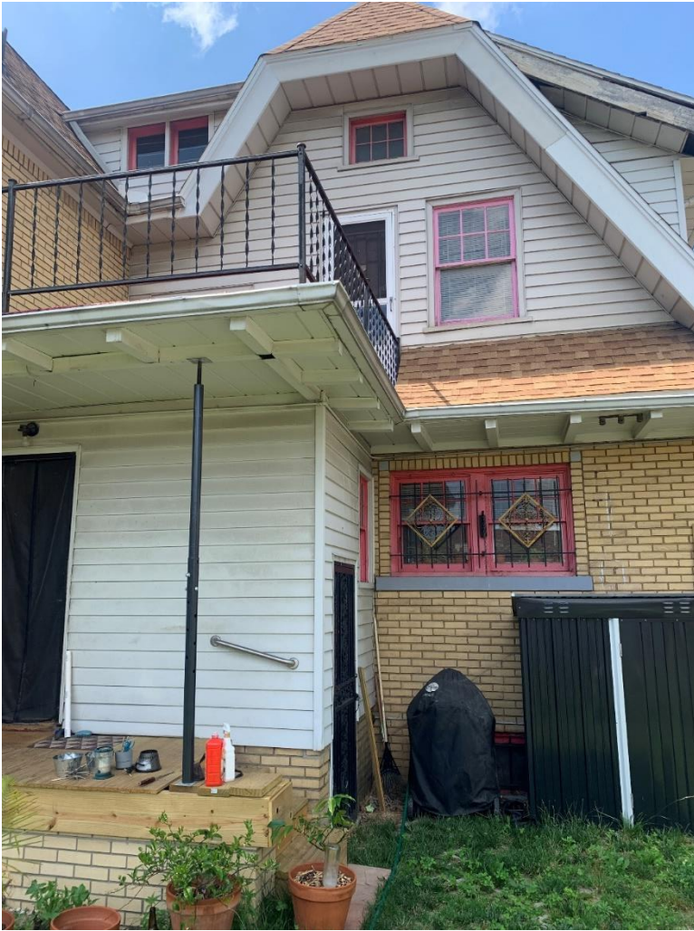
2285 Longfellow, rear. Photo provided by applicant
