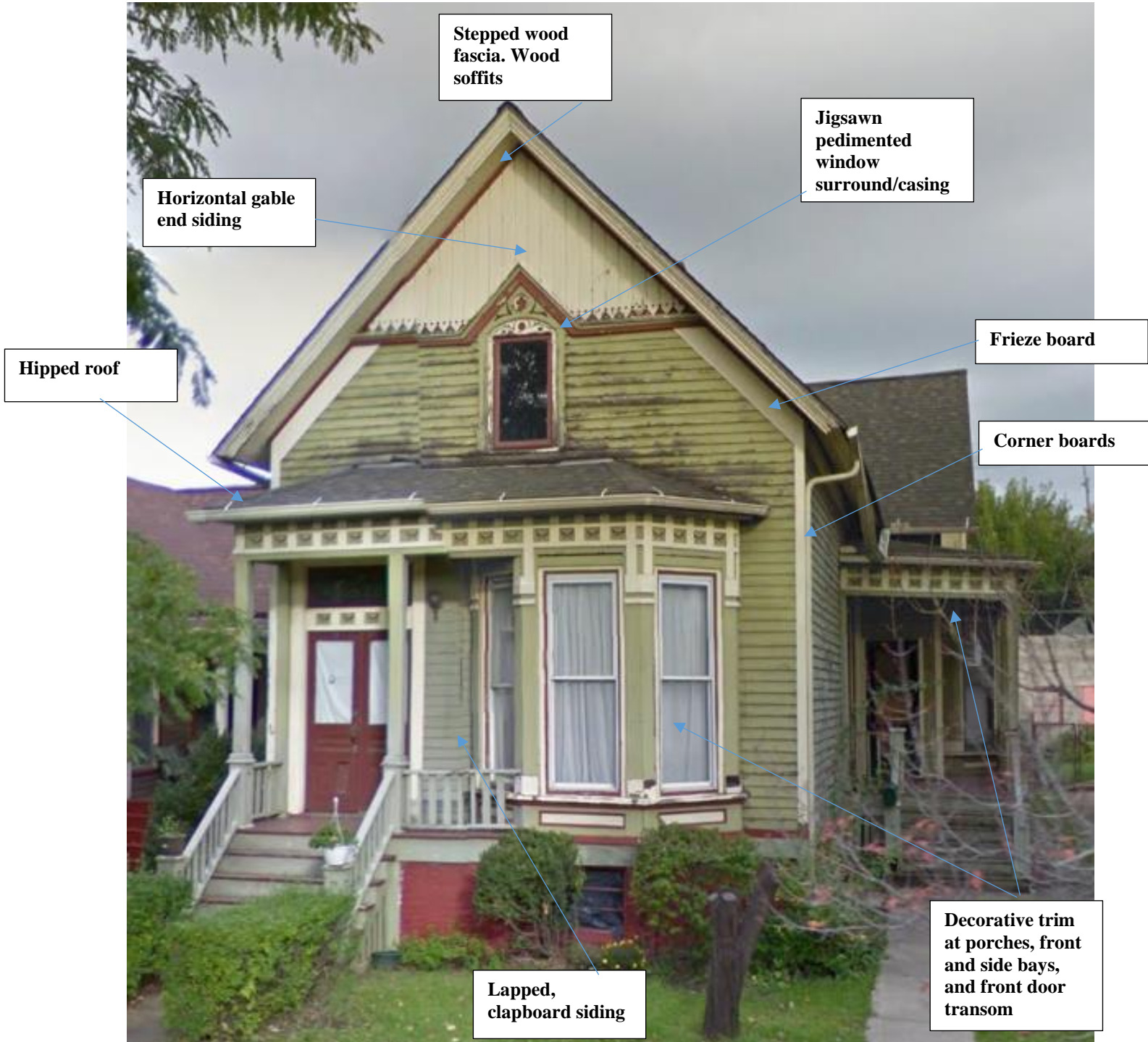
Appearance in 2016, after faux brick asphalt siding was removed. Note exposed decorative detailing at front gable end, above the front door, at the front porch roof and bay window, and at the side porch roof and bay window. Also, the front and side porch posts, piers, decking, and steps which were extant in 1983 have been replaced by this time. Source: Google Streetview
