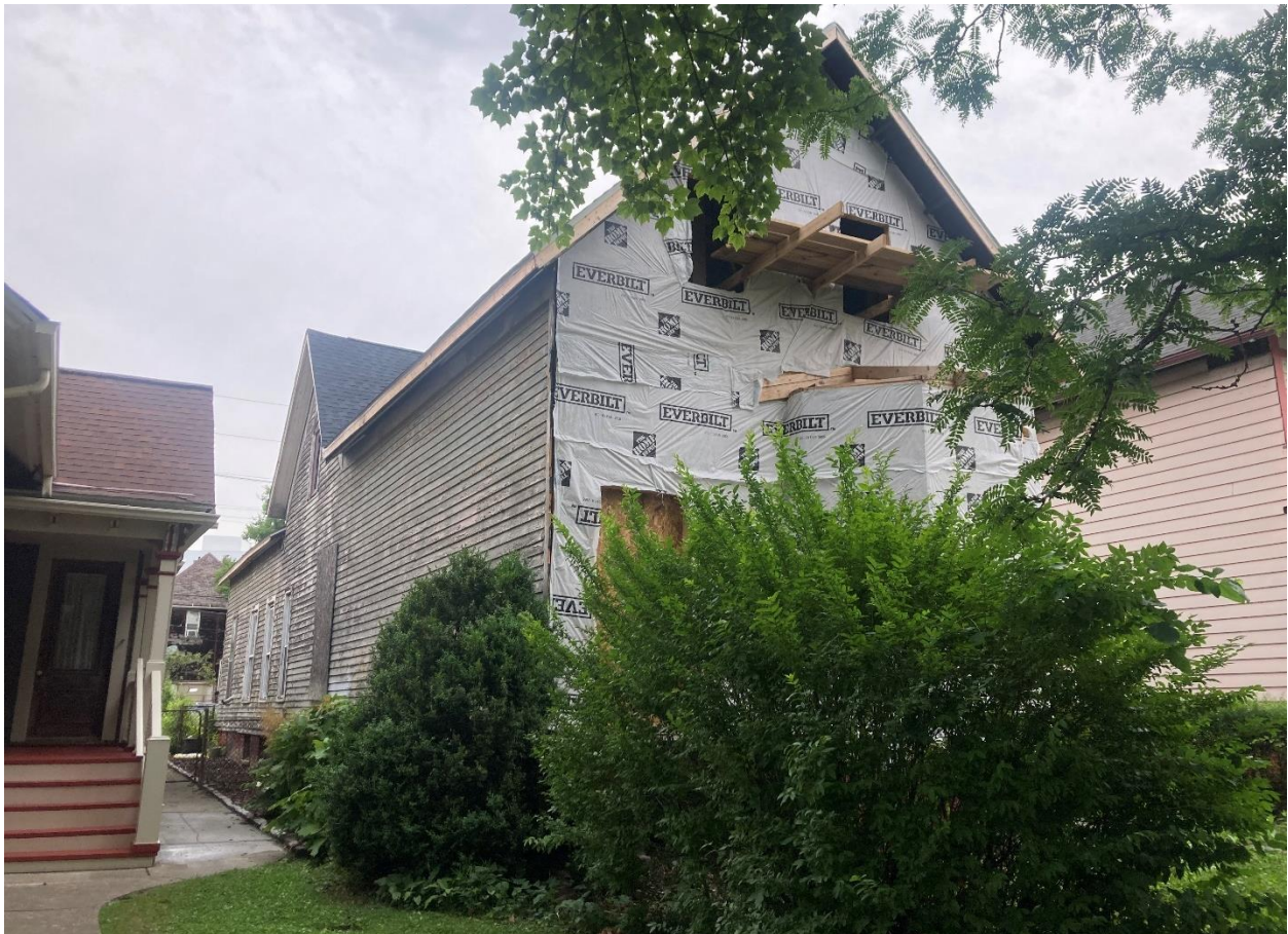
1628 Leverette, current conditions facing northeast. Staff photo taken 6/25/2024
