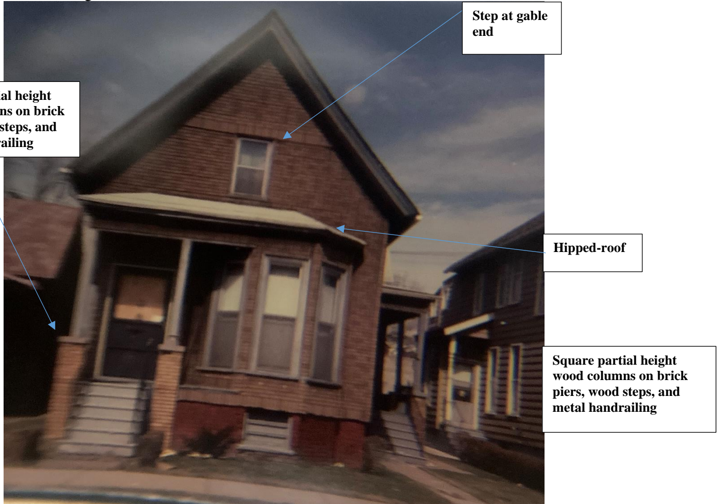
1628 Leverette, photo taken in 1983 by HDAB. Note that any exterior decorative detailing/trim is covered by the siding
