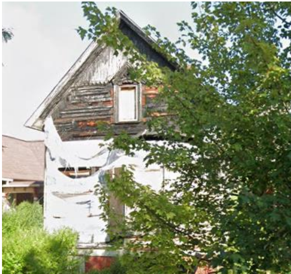
Appearance in 10/2023. Prior to unapproved work. Google Streetview
