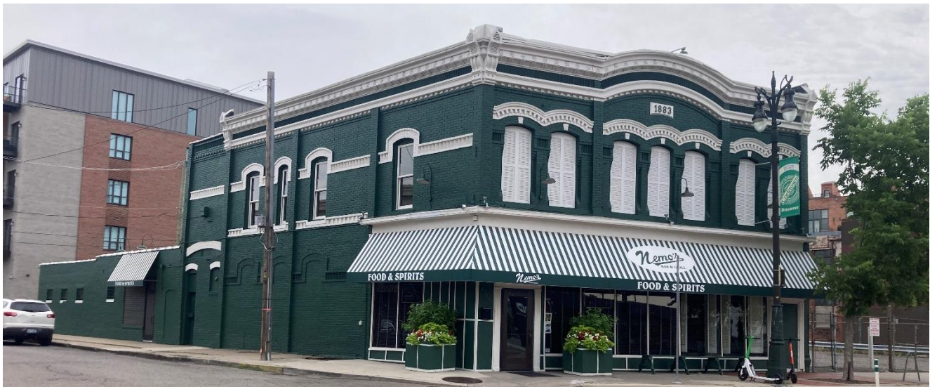
1367-1378 Michigan Avenue, facing northeast. Photo taken by staff on 6/25/2024
