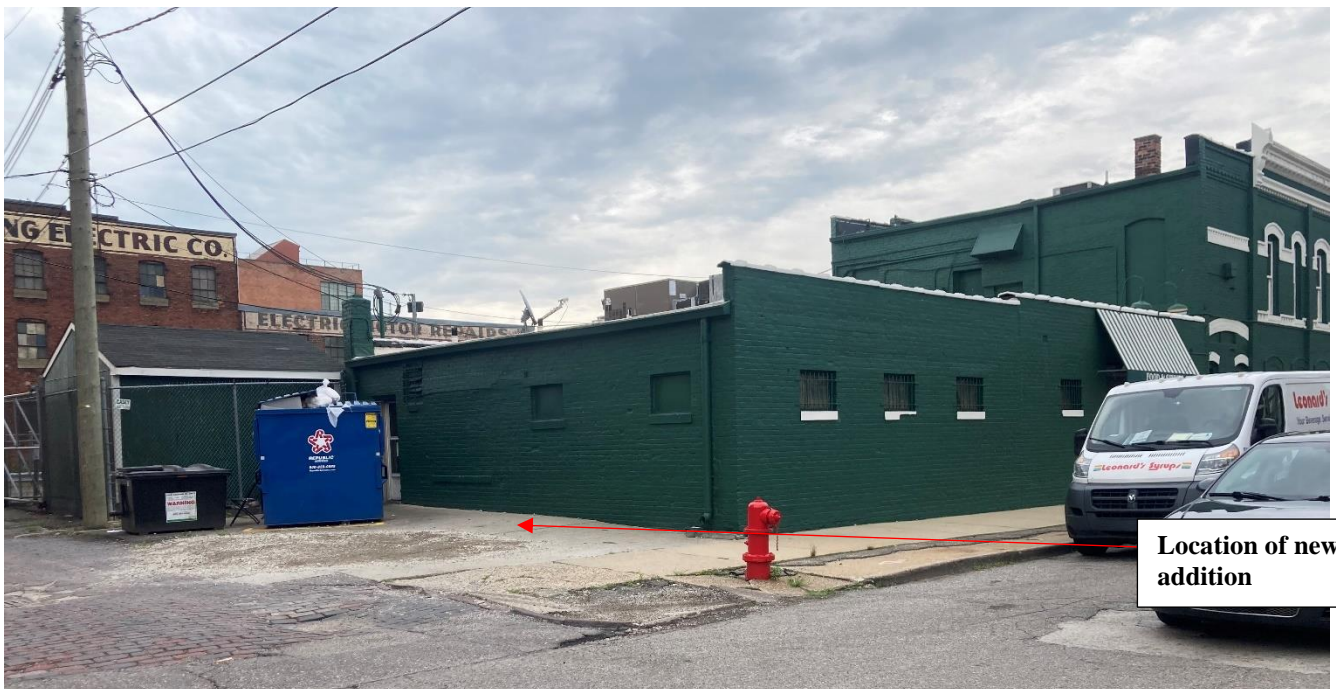
1376-1378 Michigan Avenue, facing southeast. Current conditions. Staff photo taken on 6/25/2024
