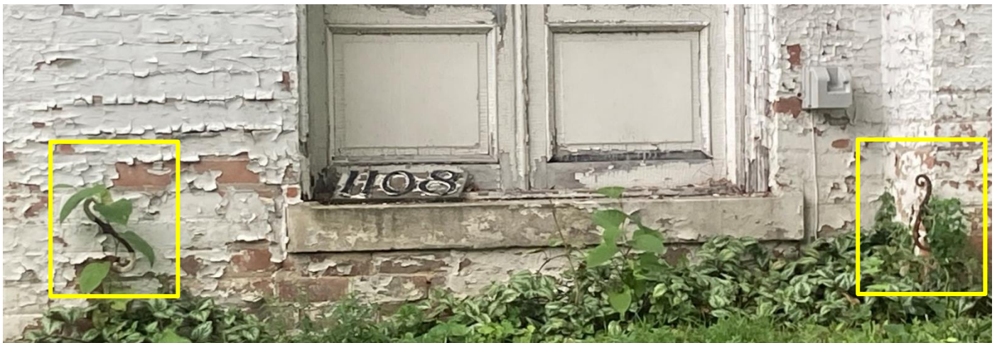
1108 Van Dyke, facing southeast, showing iron shutter dog (outlined in yellow) at west elevation Staff photo taken on 6/25/2024.
