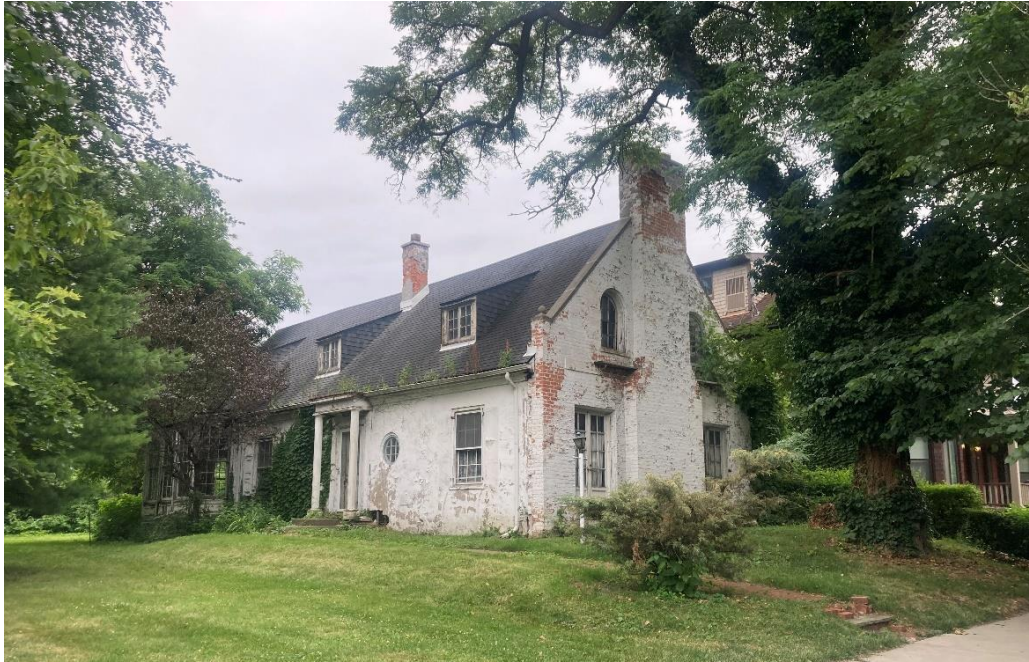
1108 Van Dyke, facing southeast showing current conditions. Staff photo taken on 6/25/2024
