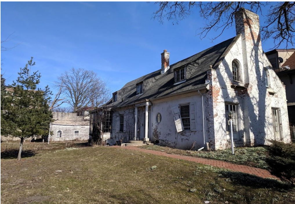
1108 Van Dyke with garage to rear. HDC staff photo taken in 2018
