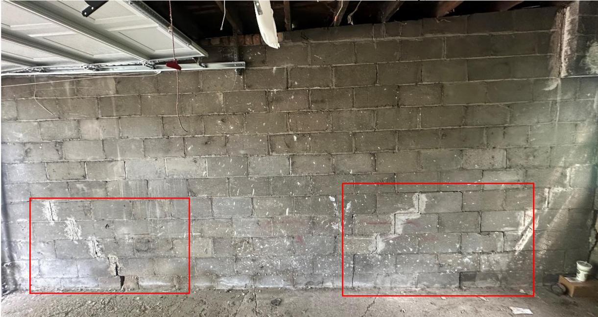
*Step crack and cracked block*
