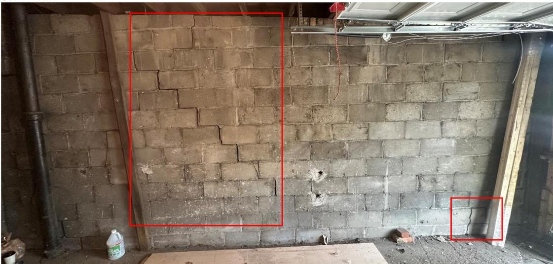
*Large step crack, broken block at top, near middle of box*
