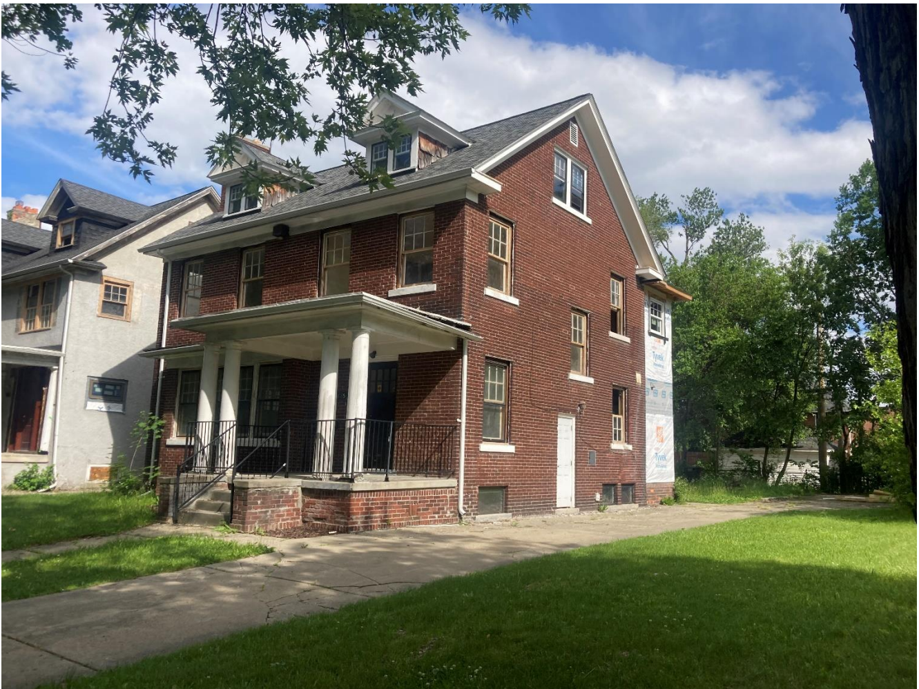
1485 Longfellow, current conditions. Facing southwest. Staff photo taken on 5/29/2024
