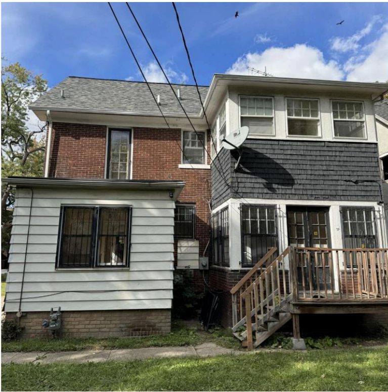
Rear of home, prior to unapproved work, facing north. Photo provided by applicant.
