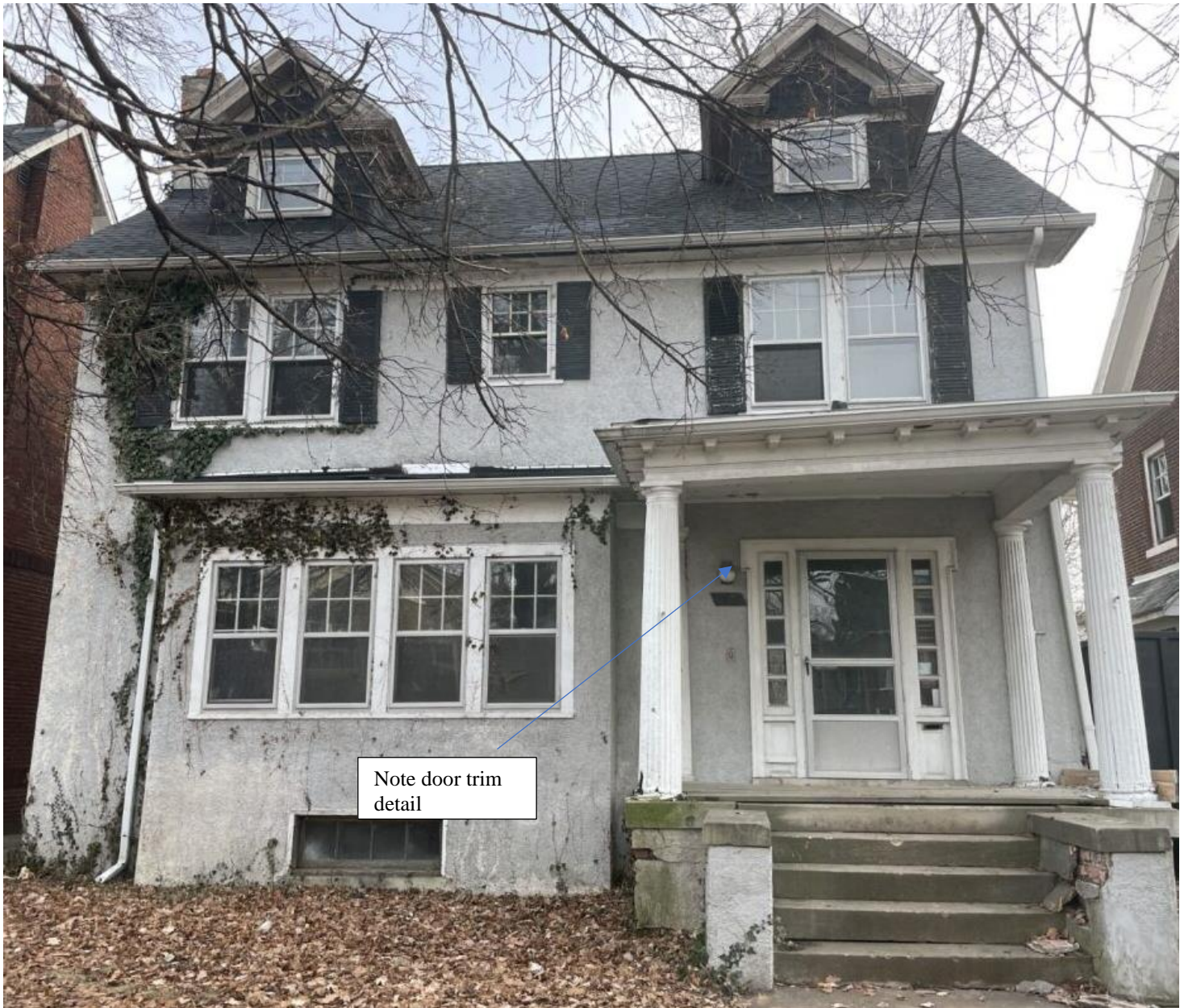
Photo of 1475 Longfellow taken by staff in 12/2023. Appearance prior to unapproved work. Note that the original character-defining porch posts, front door/sidelites and shutters remained at this time.
