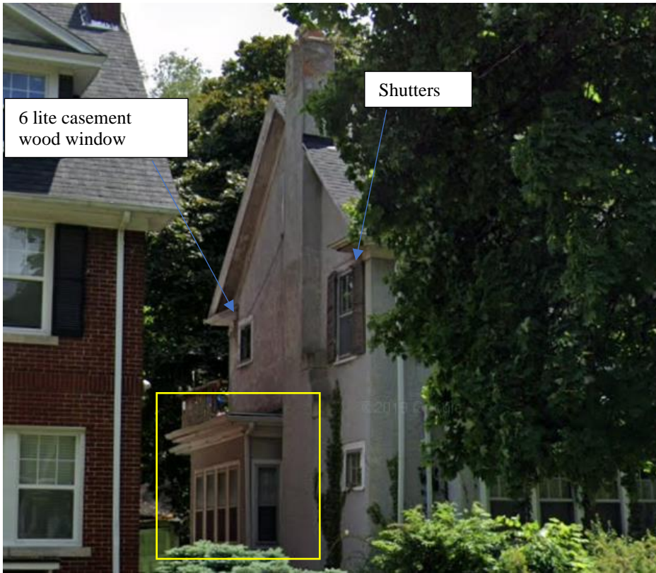
East elevation, Google Streetview, 2022. Note original windows, shutters at second story, and projecting sunroof bay at first story (outlined in yellow). This bay also extended to the building's rear elevation
