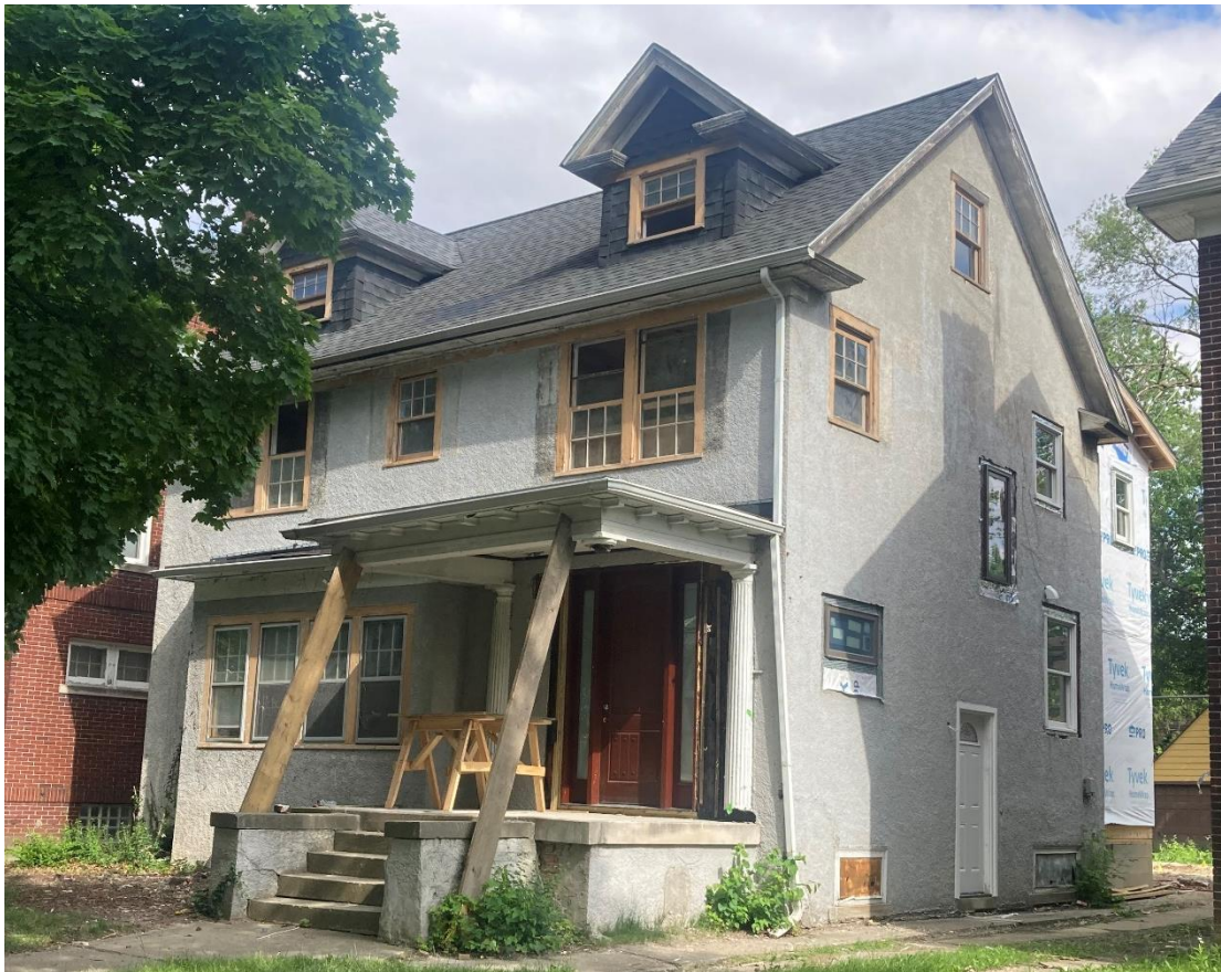
1475 Longfellow, staff photo taken on 5/29/2024. Facing southeast.
