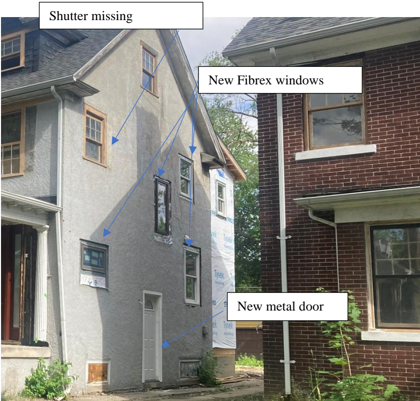
West elevation, staff photo taken on 5/29/2024. Note that shutters and the original wood door at the first story has been replaced with a metal door with a fanlight vision panel. Also, note four new windows have been added
