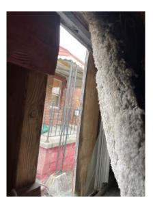
Site Photo 4, by Applicant, showing interior garage door window slider with wood framing and metal sash, which is proposed for replacement with a vinyl slider.
