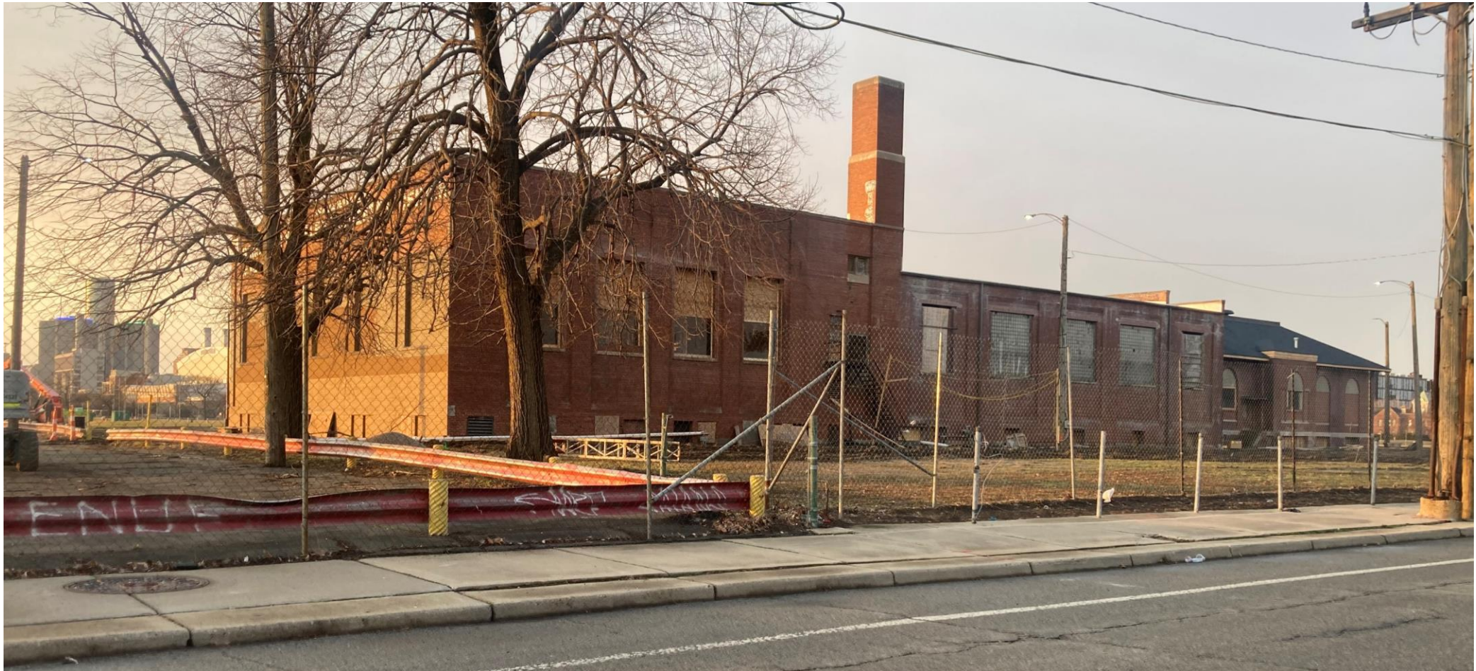
FACING SOUTHWEST. 1929 ADDITION IN THE FOREGROUND
