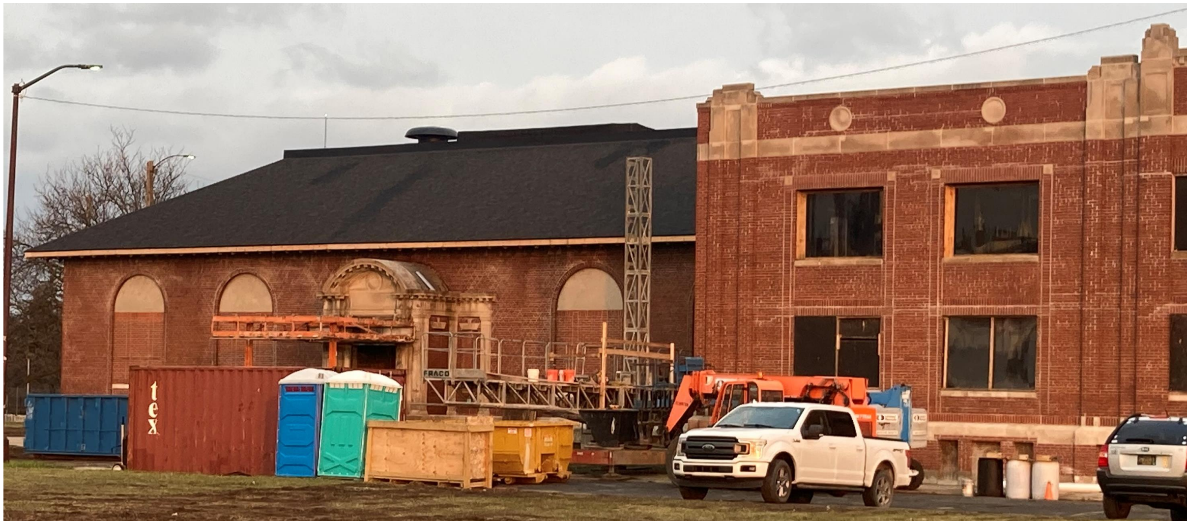
FACING NORTHWEST, SHOWING THE ORIGINAL 1917 LIBRARY WING
