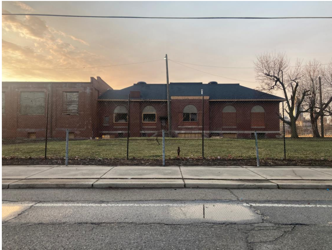
FACING SOUTH, TOWARDS ORIGINAL LIBRARY WING
