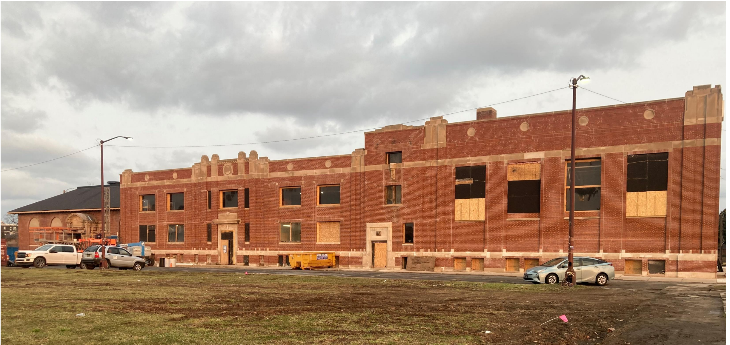
FACING NORTHWEST, SHOWING 1929 ADDITION IN THE FOREGROUND
