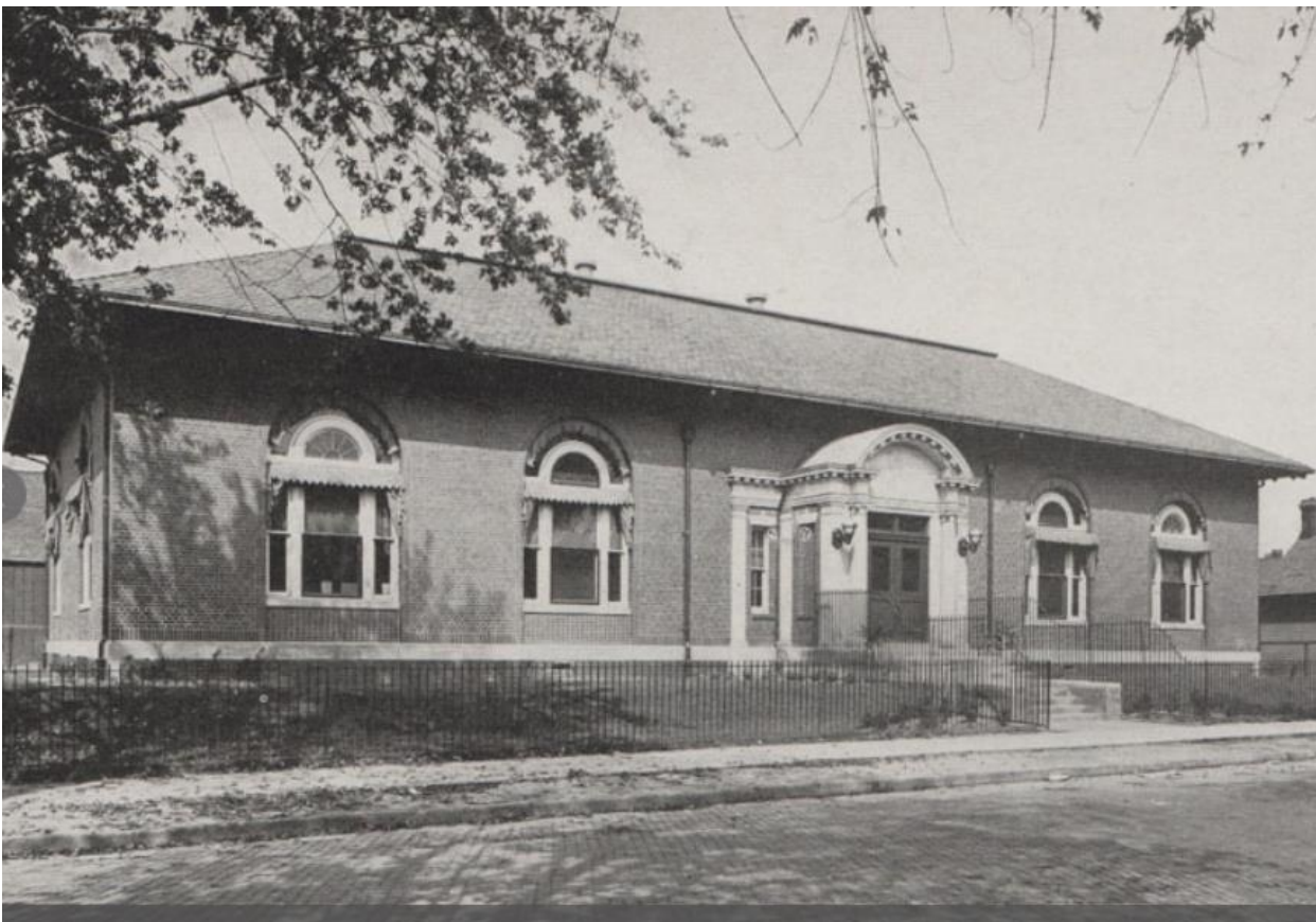
Ginsburg Library, ca. 1920. Note the projecting, arched-roofed primary entrance
