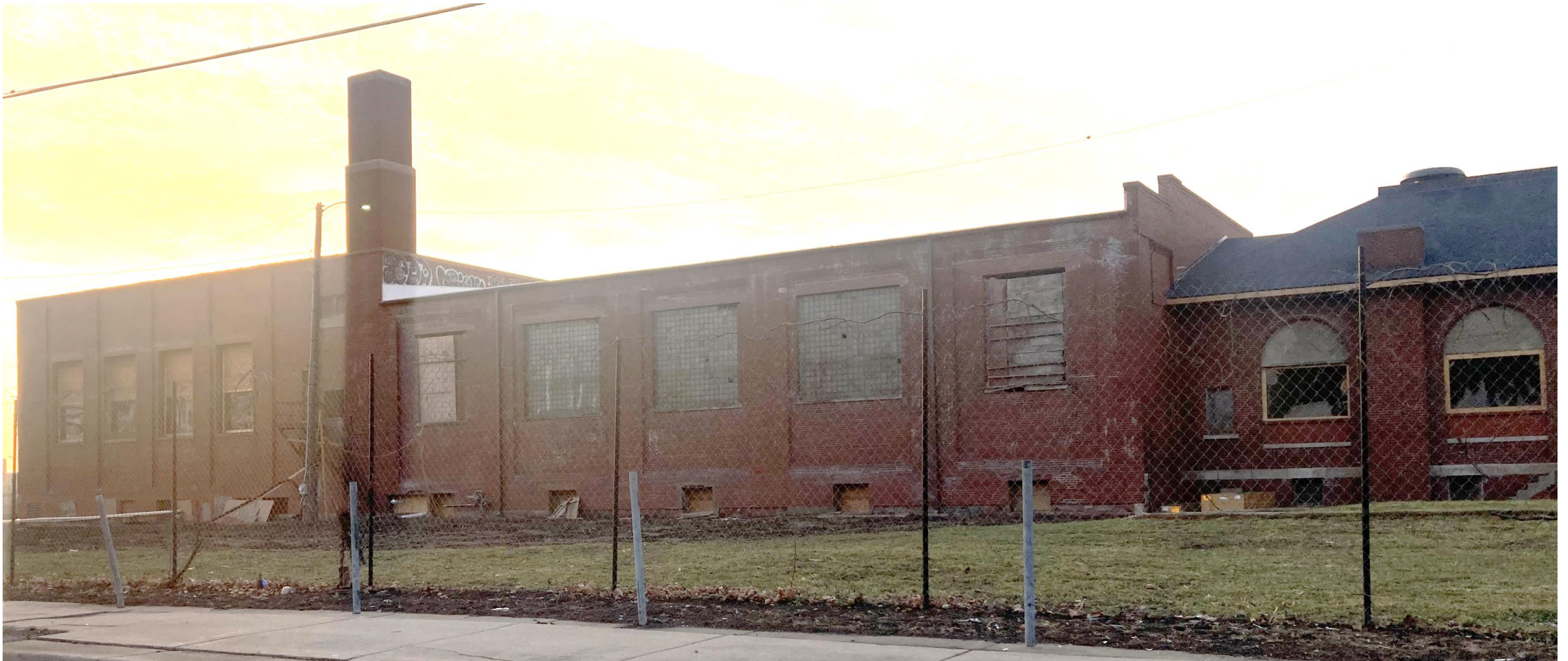
FACING SOUTHEAST, TOWARDS GLASS BLOCK WINDOWS AT 1929 ADDITION'S NORTH ELEVATION
