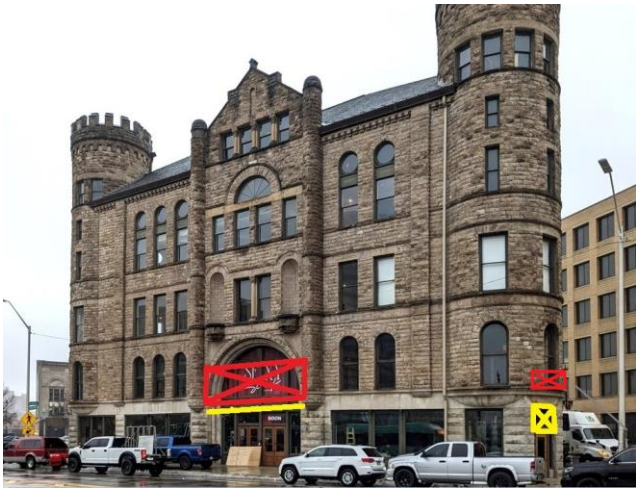
Approximate location of Grand River (southwest) façade and east corner signs (red) and awnings (yellow). Sketch by staff.
