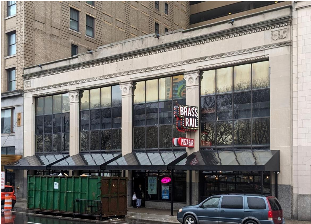
The subject property viewed from Grand Circus Park across the street. The Brass Rail sign depicted is a violation. January 2024 photo by staff.
