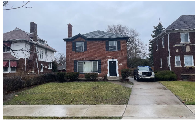
Site Photo 3, by Staff January 3, 2024 showing new roof, painted soffits, and new front door.
