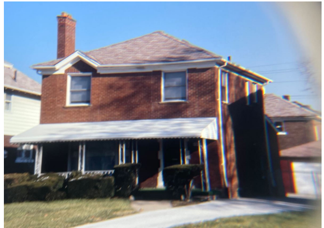
Designation photo 1999: (west) front elevation, showing existing garage in the backyard, porch railing and awning, original 1/1 windows without shutters, and wood fascia and soffits and wood door.
