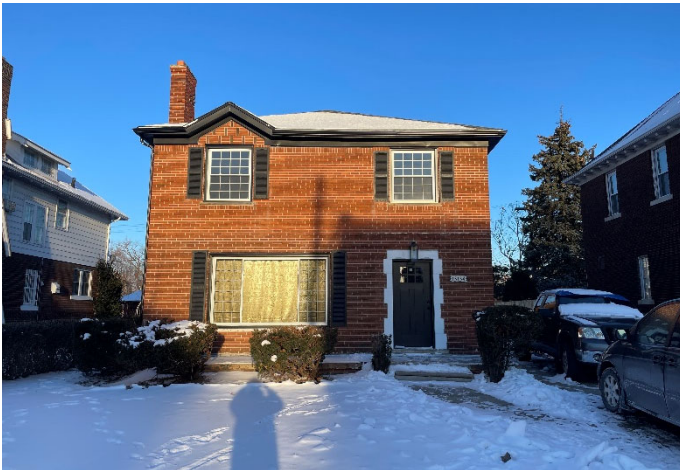
Site Photo 1, by Staff January 17, 2024: (West) front elevation.
