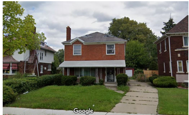
Site Photo 4, by Google Streetview Sept 2023 showing previous conditions: windows, porch awning and roof.
