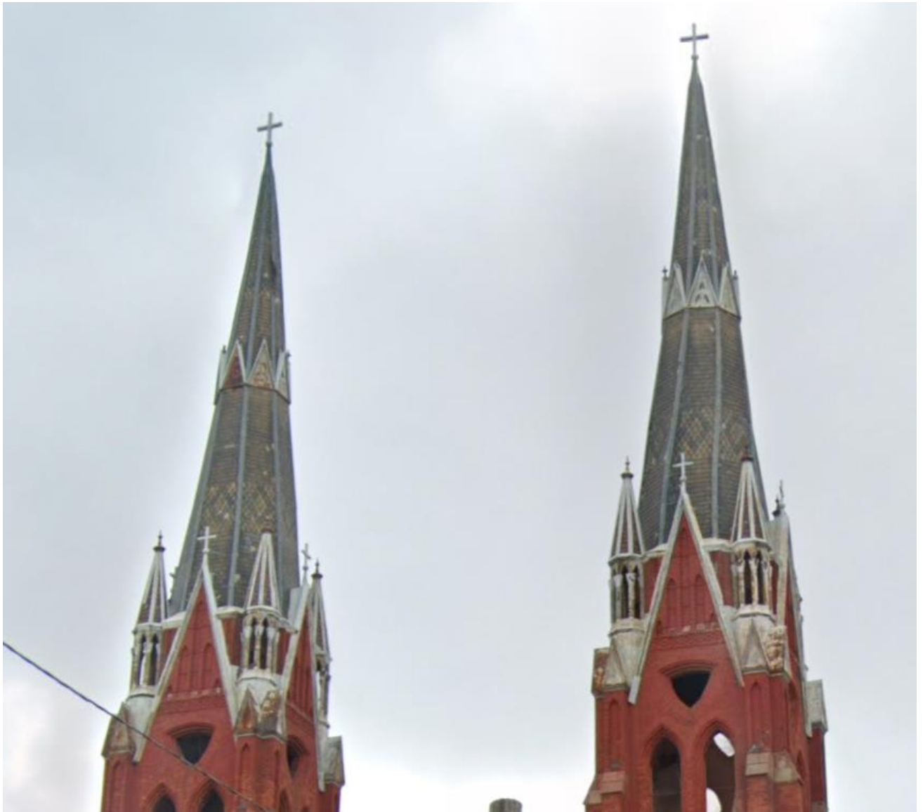
Google Streeview, August 2018, prior to steeple repair
