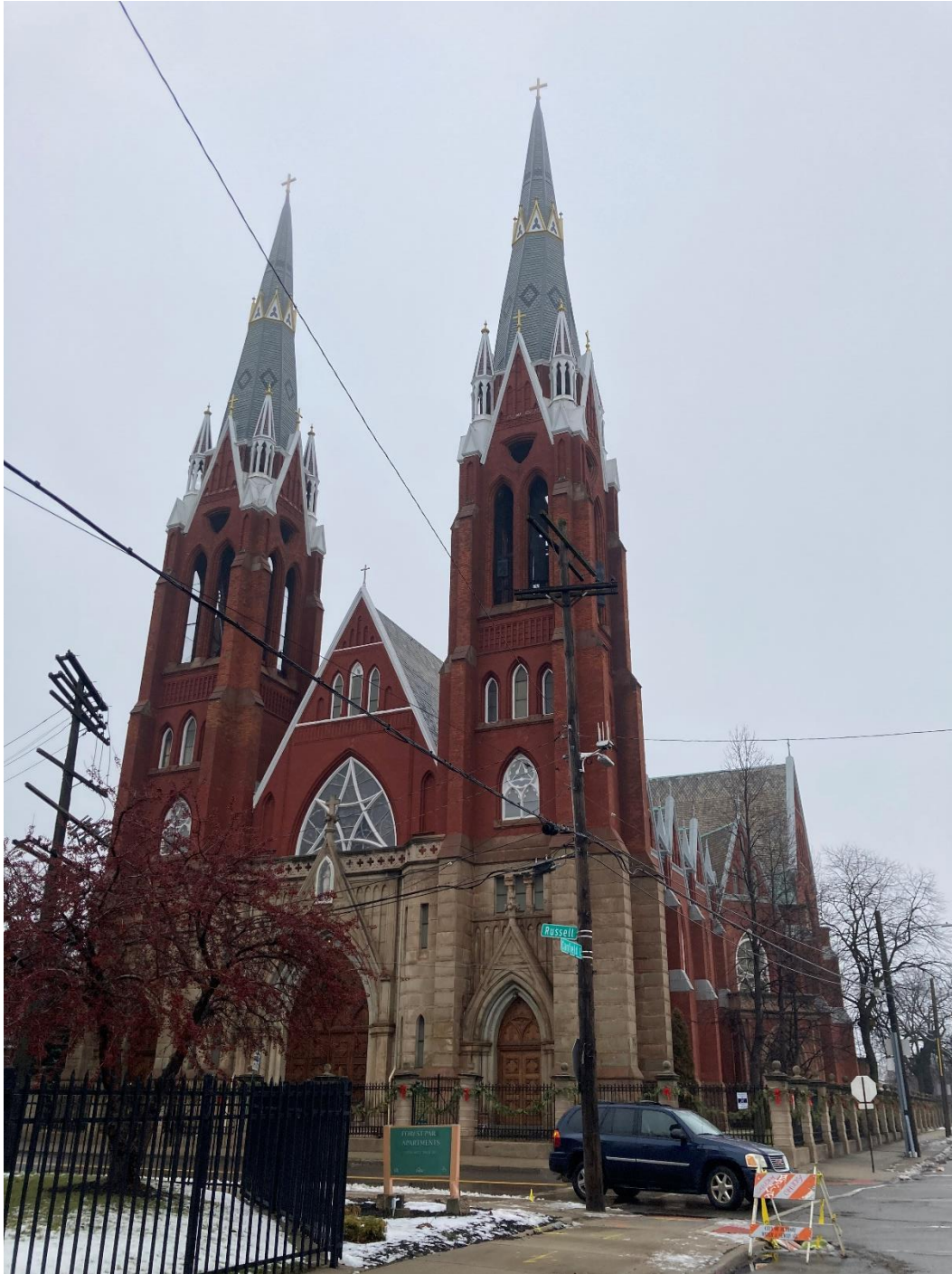
Current conditions, facing northeast showing primary façade. Staff photo taken 1/25/2024
