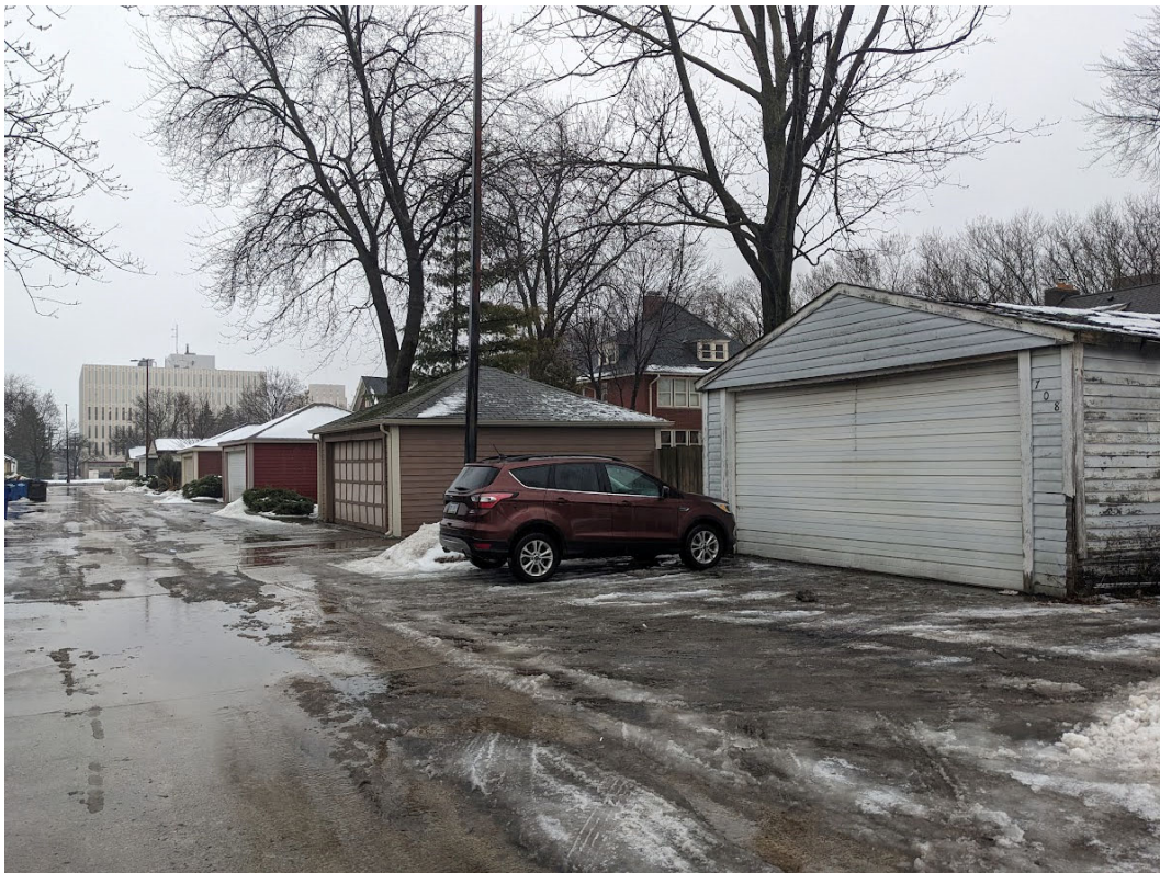
View east in alley/service drive. Some of these garages are historic reproductions that were erected during the urban renewal activities that included the formation of the historic district. Subject garage at 708 Pallister is at right. Staff photo, January 24, 2024.
