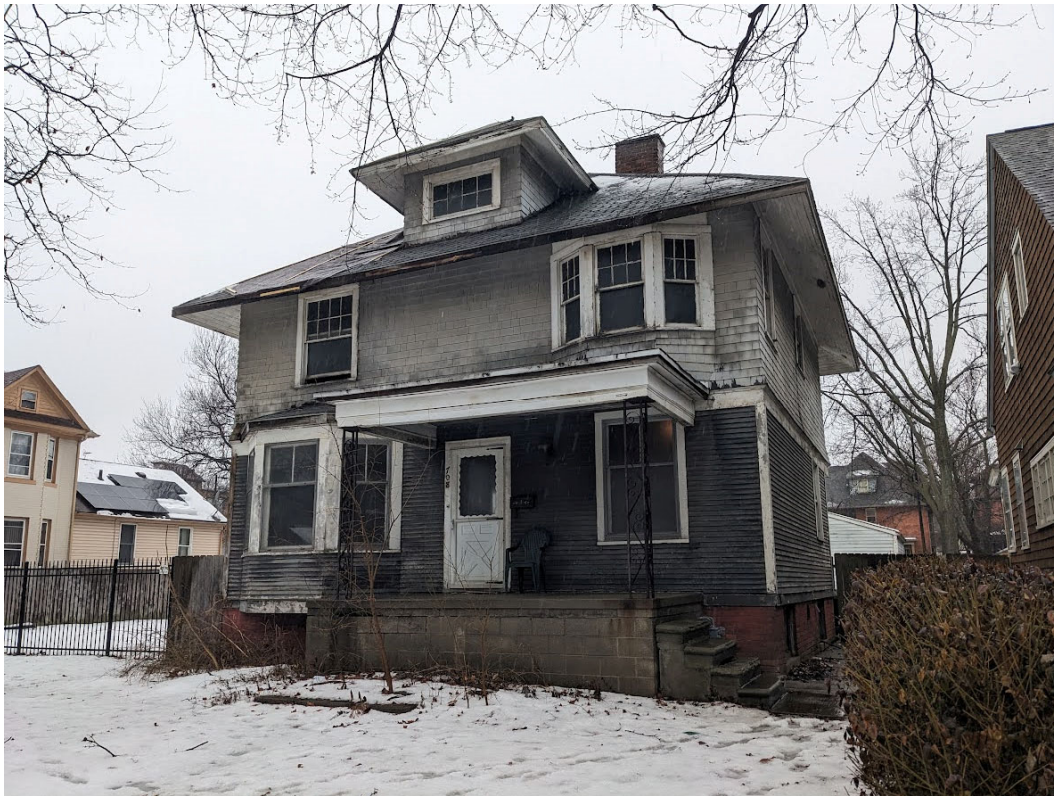
View of 708 Pallister, looking northwest from the sidewalk. Staff photo, January 24, 2024.
