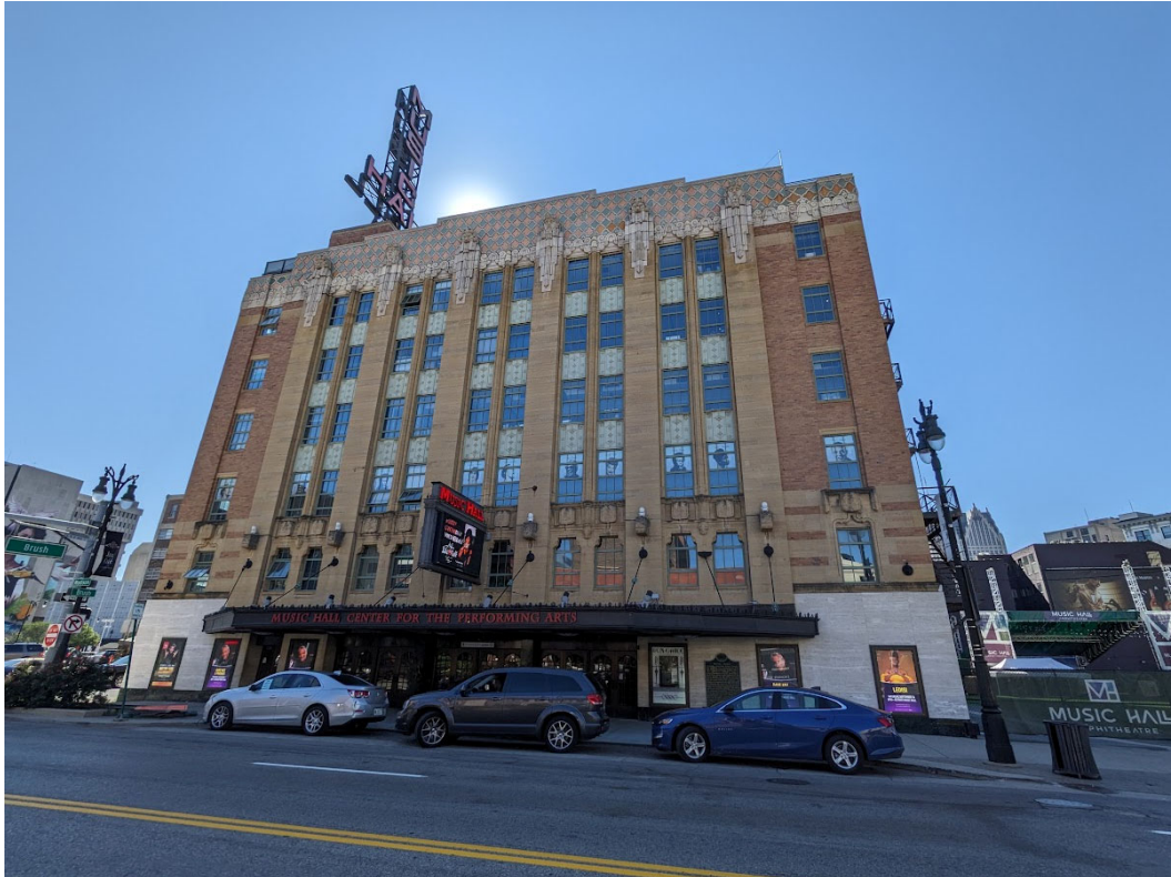
View of the Music Hall (350 Madison), looking towards the south. Development site for the new building/addition is visible at the right in this image, across an intervening alley. Staff photo, September 1, 2023.
