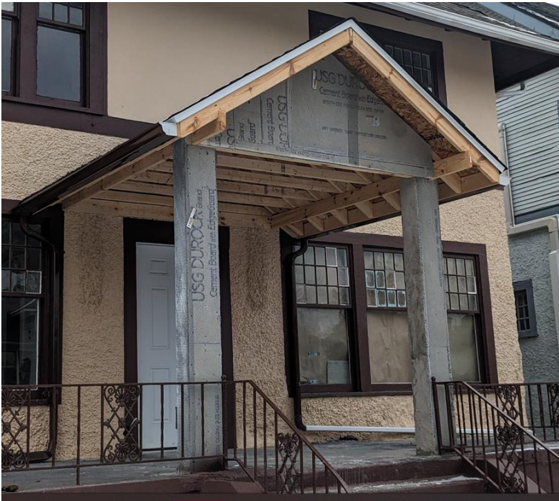
“After” photo of porch roof. November 2023 photo by staff.
