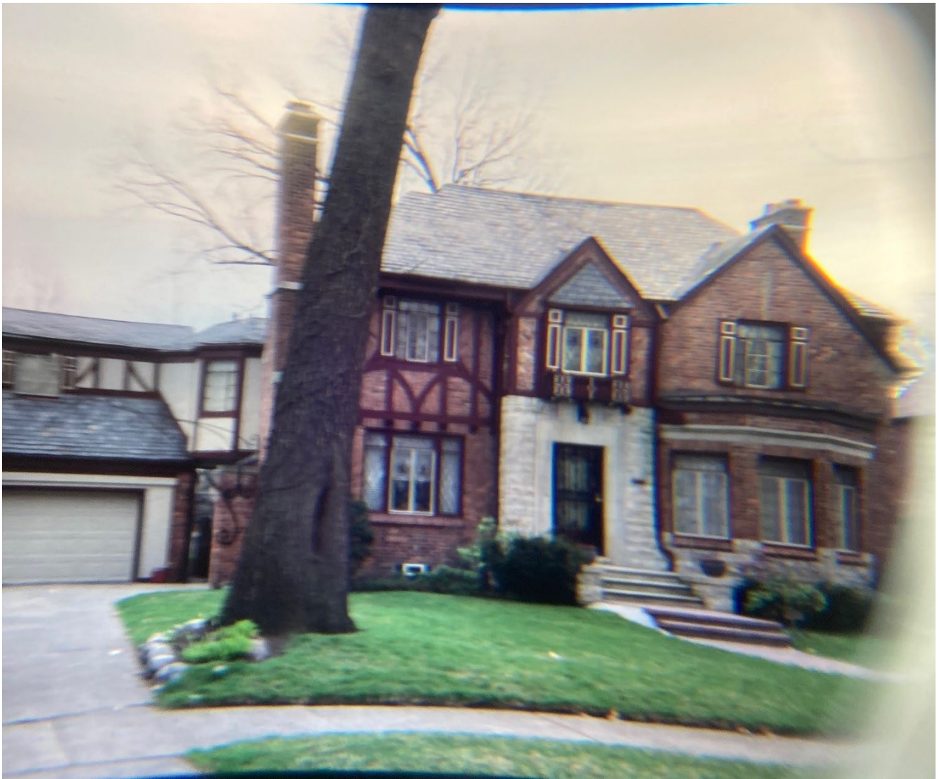
Figure 2: 2002 designation photograph of 19650 Canterbury showing the original slate roof. HDAB
