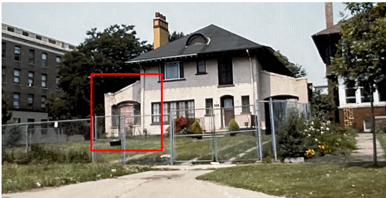
3964 W. Lafayette, designation slide, wing proposed for rehabilitation
