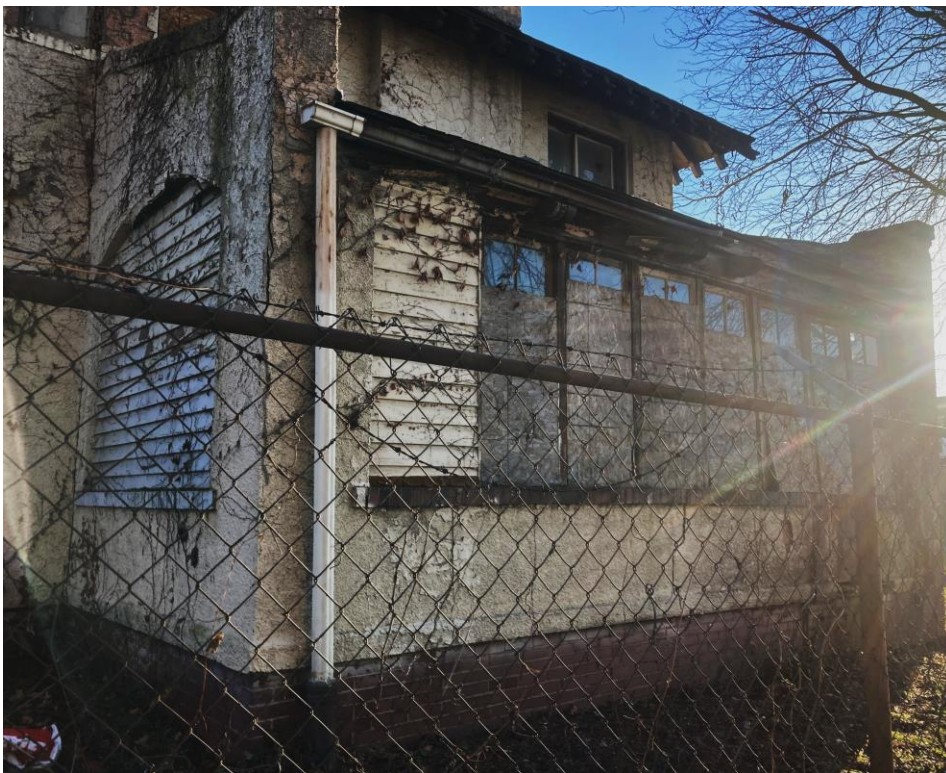
Staff photo, facing southeast showing wing proposed for rehabilitation, taken 12/8/2023
