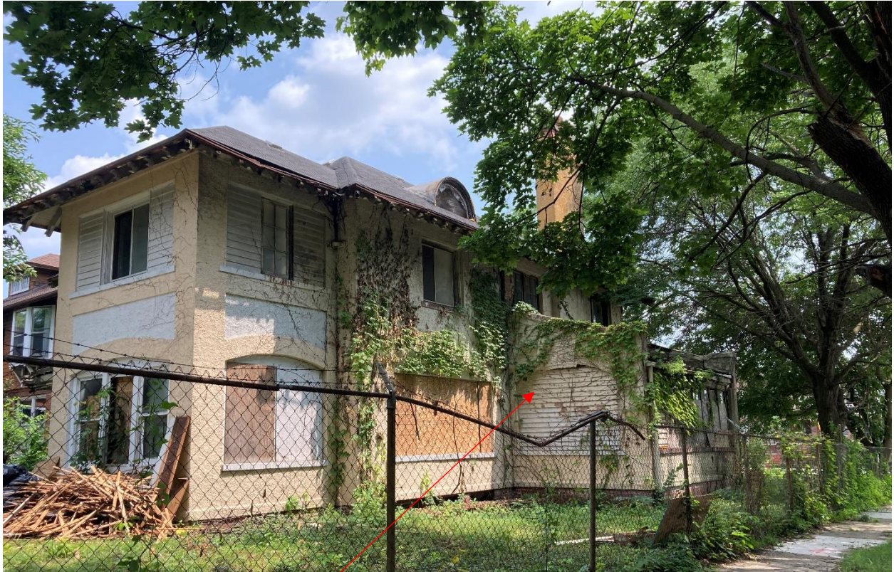
Facing southeast. The north wall shown here will be retained
