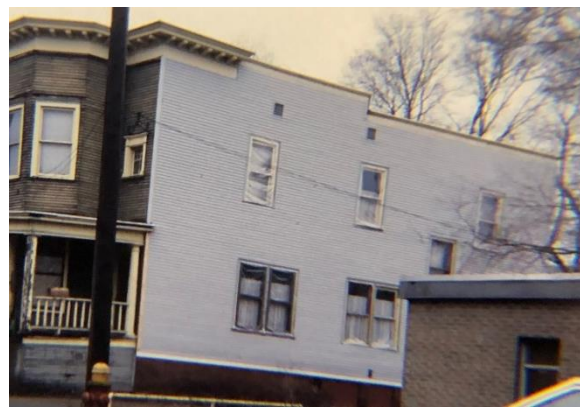
North elevation, designation photo, 1984.
