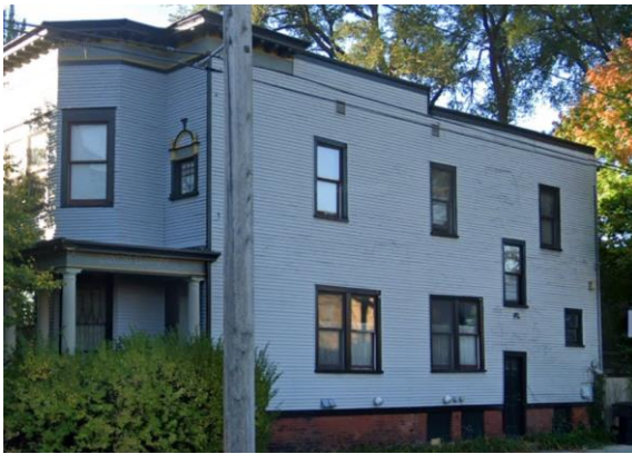
North elevation, Google street view, October 2020.
