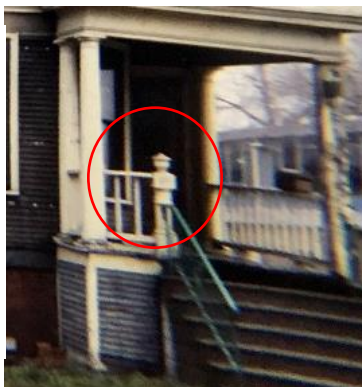
Designation photo, 1984. Circled is the corner post that was to be reinstalled upon installation of a new wood porch and stair railing. An identical post was similarly in place at the adjacent porch.
