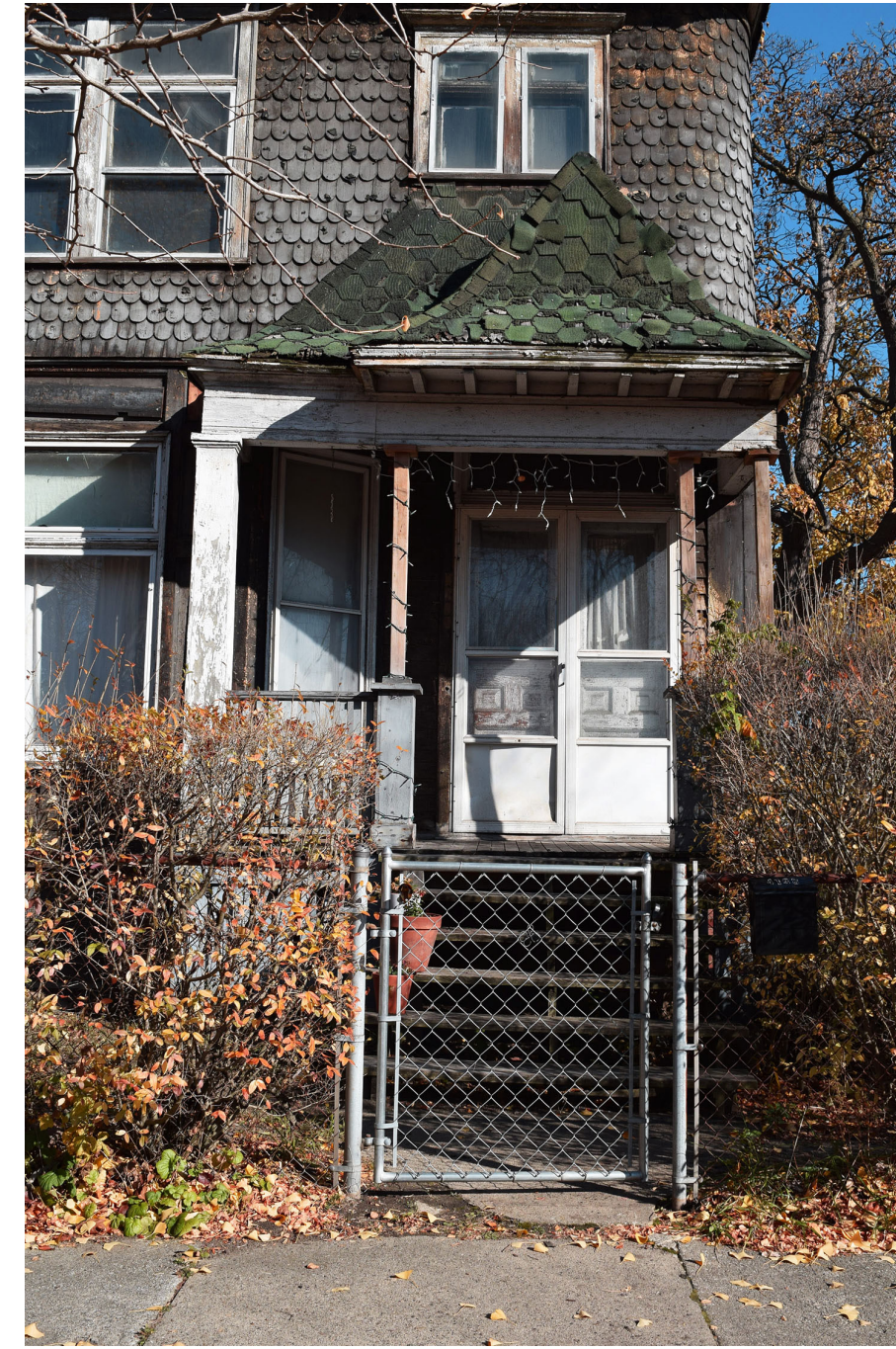
2 FRONT PORCH (SOUTHWEST)
