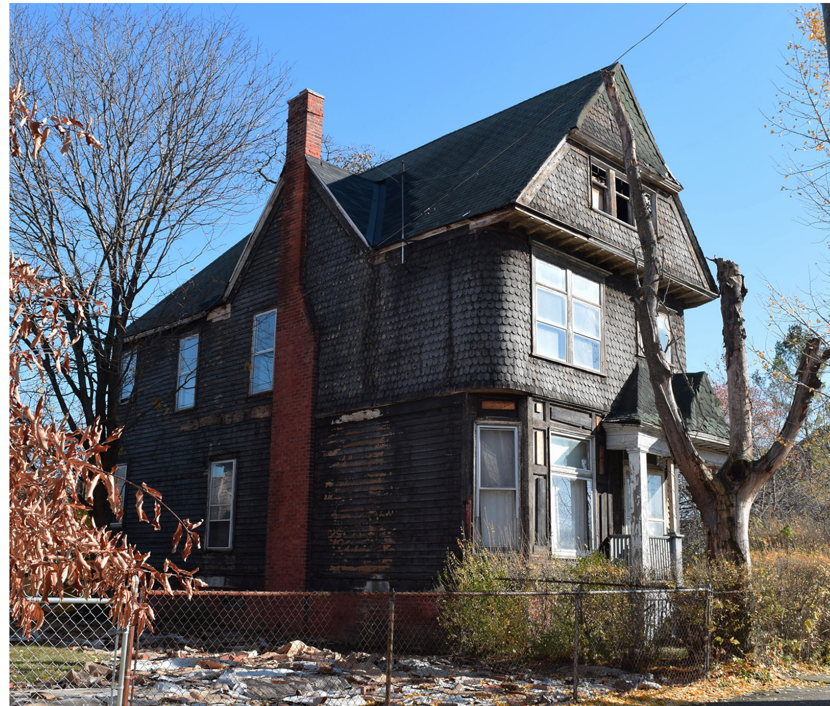
5 SIDE FAÇADE (NORTHWEST)
