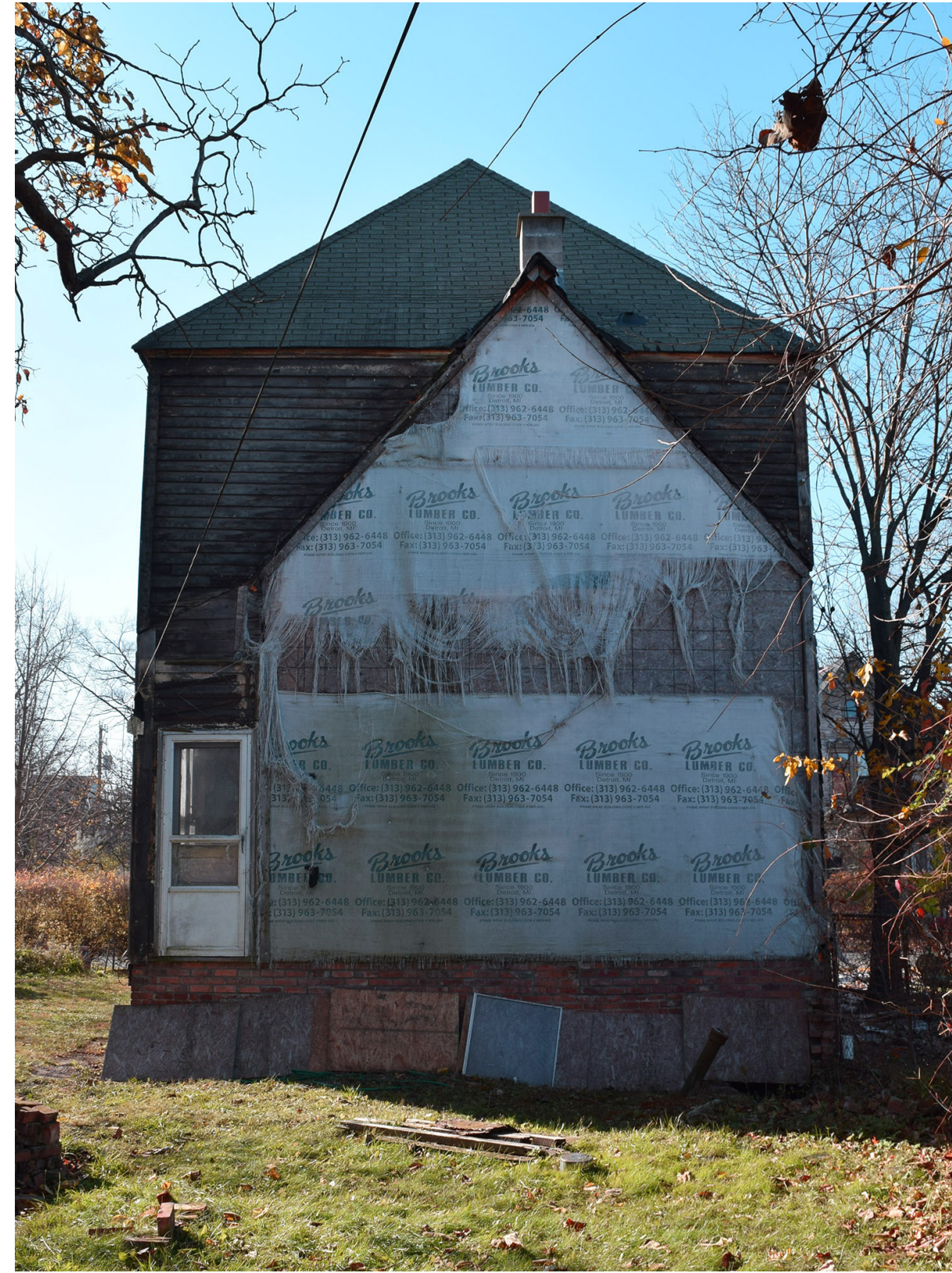
3 REAR FAÇADE (NORTHEAST)
