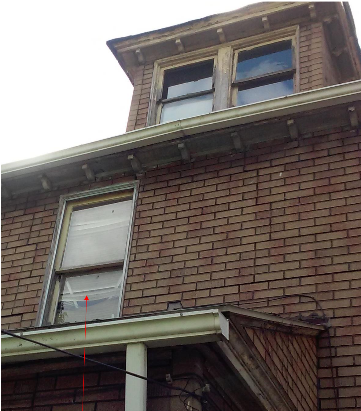
Rear elevation, second story
