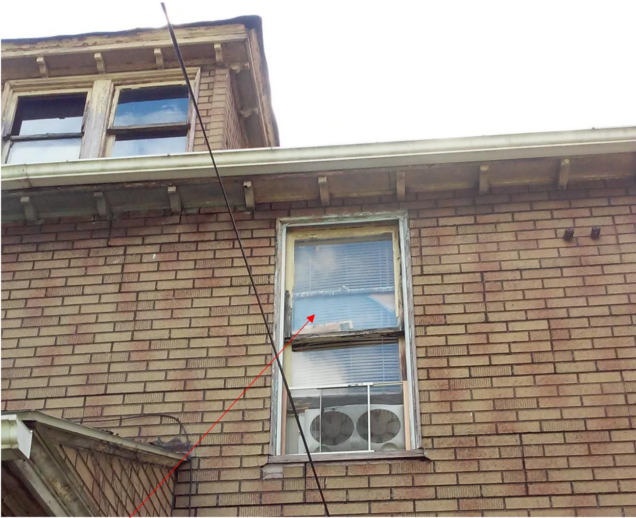
Rear elevation, second story
