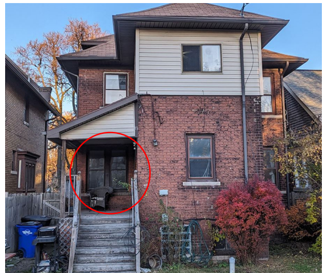
Site Photo 4, by applicant showing location of rear window proposed to be replaced by casements.
