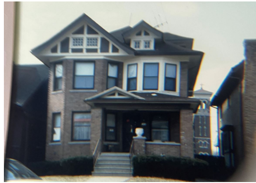
Site Photo 2, Designation Photo March 1983: (east) front elevation.
