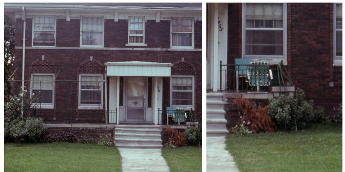
Photos 4-5, from 1974 Designation Photo: front porch detail with brick pier end posts, metal railing, concrete coping with concrete steps, brick clad walls and wingwalls.
