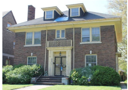
Photo 7, by Facebook Detroit Area Historic group (date unknown, showing a Juliette balcony railing and entrance façade.
