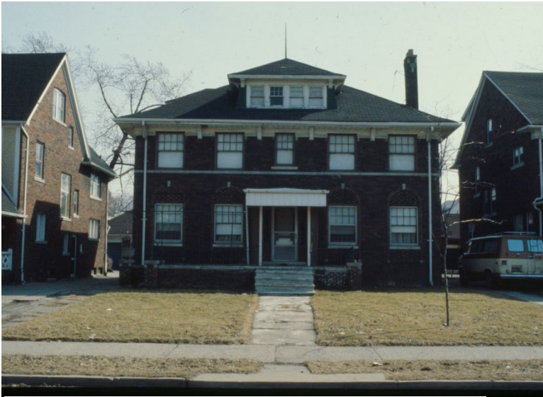
Photo 3, Historic photo, by HDAB 1980: (Northwest) front elevation.
