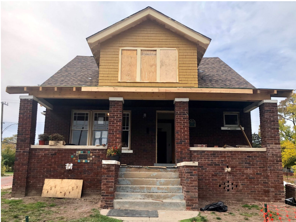
East elevation. Staff photo, October 25, 2023.
