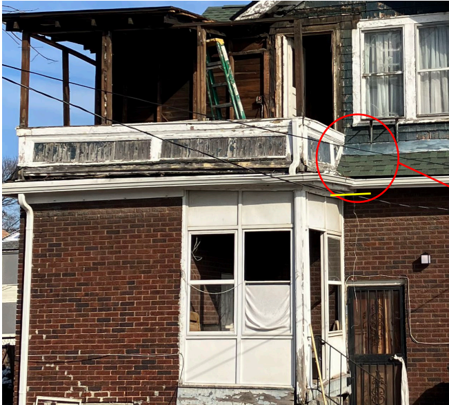
Above: Undated applicant photo documenting demolition of the second floor rear porch. Note that the top of the knee wall is in line with the top of the first row of wood shingles.
