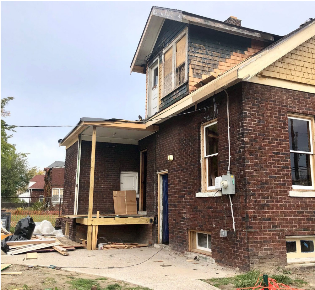
Rear elevation elevation, looking north. Staff photo, October 25, 2023.
