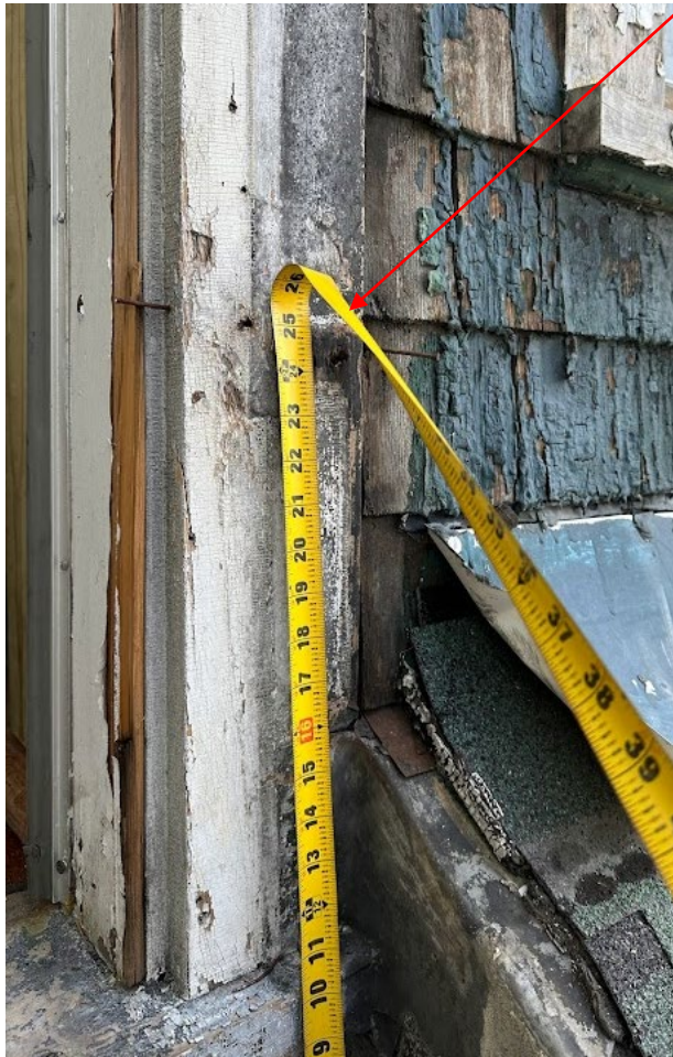
Below: Recent applicant photo. The tape measure confirms an approximate 25-inch height of former railing/knee wall.
