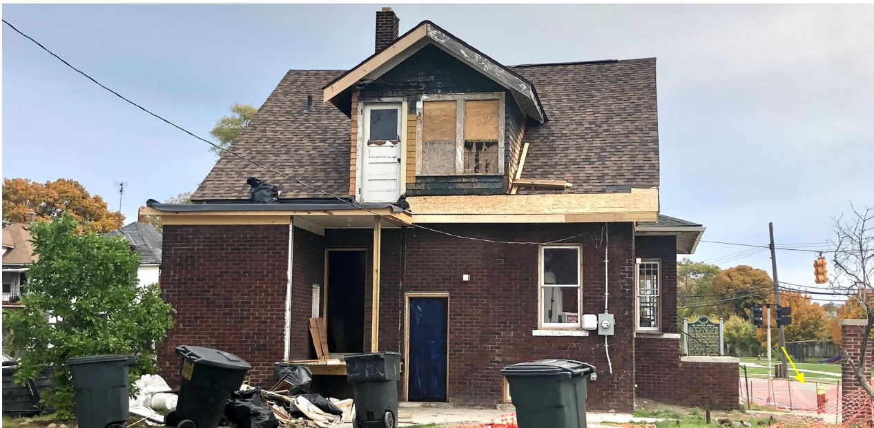
Rear-west elevation. Staff photo, October 25, 2023.
