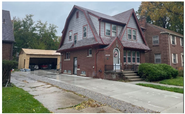
Site Photo 2, by Staff October 19, 2023 showing new garage and driveway.
