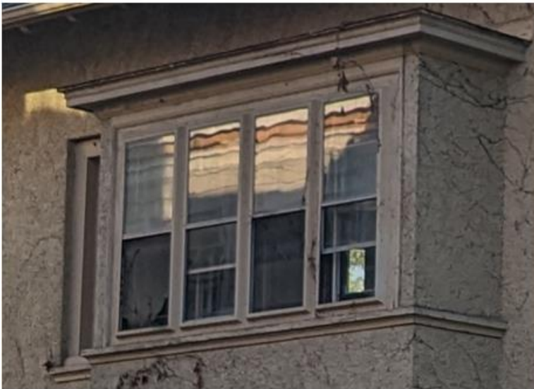
Left: Box bay with wood, one-over-one sash windows (not readily visible due to glare from storm windows). Right: Wood window, possibly a fixed or hopper window (typical of both). October 2023 photos by staff.
