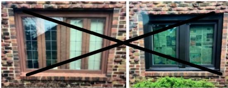
Before (left) and after (right) examples of aluminum cladding provided by the applicant. Note that the proposed color is white rather than the black shown.
